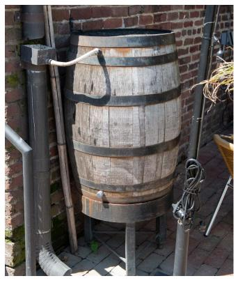
There are two types of rainwater harvesting practices that property owners can consider installing – rain barrels and cisterns. The practices operate similarly, but cisterns are much larger than rain barrels and can store hundreds of gallons of water. The practice must capture runoff for reuse from at least the first one inch of a rain storm to be eligible for credit.
