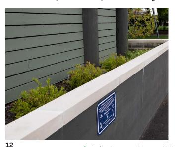
limited space available for stormwater treatment by placing a soil filter in a container located above ground or at grade in landscaping areas (often between buildings and roadways). The planter box is typically contained in a precast or cast-inplace concrete vault and has an underdrain.
