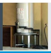
Elevating key components associated with a property's heating, ventilation, and air conditioning (HVAC) system, along with other major appliances such as washers, dryers, and hot water heaters from basement areas to a higher floor or the attic is the best way to mitigate against future flood damage.
