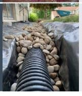
The purpose of a French drain is to direct surface run off water and groundwater away from the home's foundation. These types of drains are ideal because they reduce pressure and remove excess moisture from the soil by collecting surface water and groundwater.
