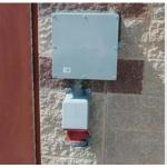
In homes provided with a flanged connection (often called a "Quick Connect") to connect a temporary generator to the main electrical panel, the flanged connection should be placed above the required flood elevation in a place that allows a generator to be brought onto the property, quickly connected to the property, and safely refueled when needed.
