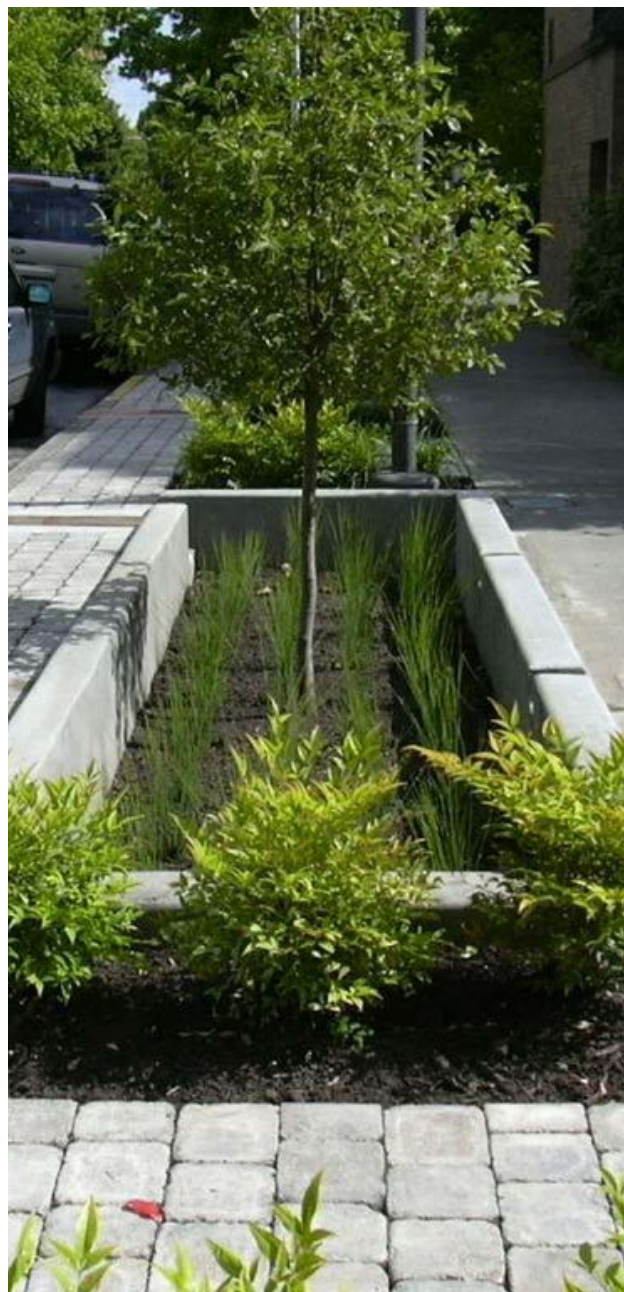
URBAN BIORETENTION TREE WELL, PORTLAND, OREGON
