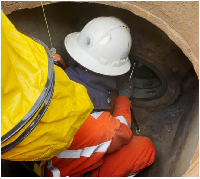
Engineer Altan Erginkoc observed the check valve installation using on-call contractor at East Mason Avenue and Dewitt Avenue on Nov. 30
