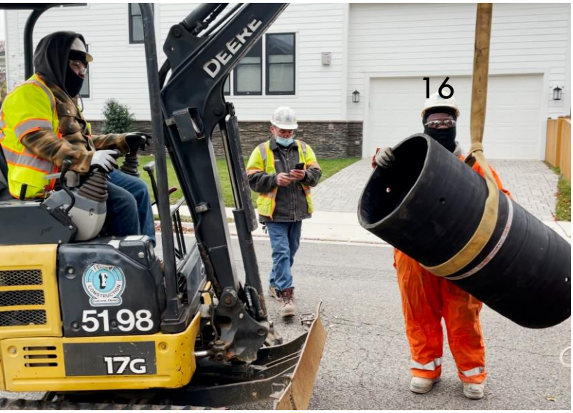
Engineer Altan Erginkoc observed the check valve installation using on-call contractor at East Mason Avenue and Dewitt Avenue on Nov. 30
