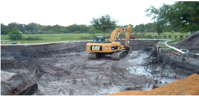
Excavate Soil in Saturated Conditions
