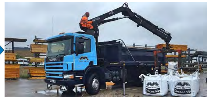
Load Watertight Bags onto Truck
