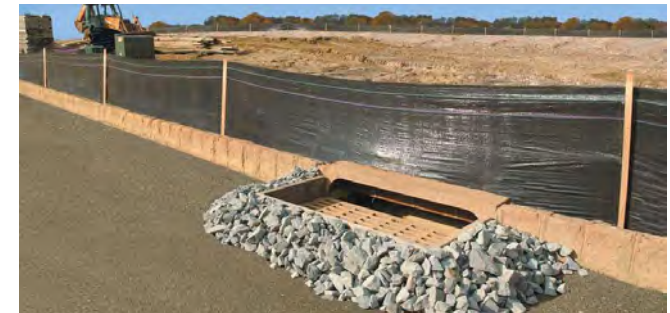
Erosion & Sediment Control
