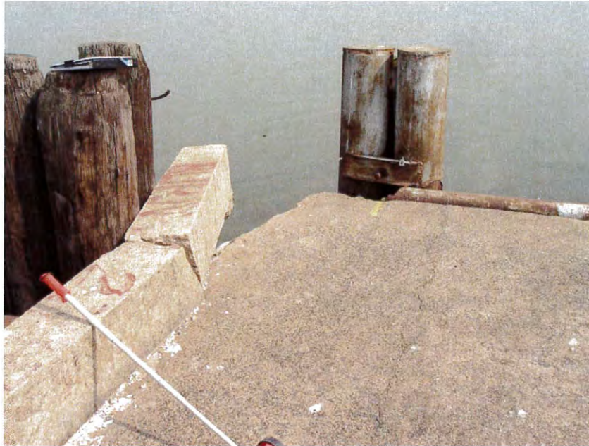
Photo 3-14 – Damaged Curb at Northeast Corner
