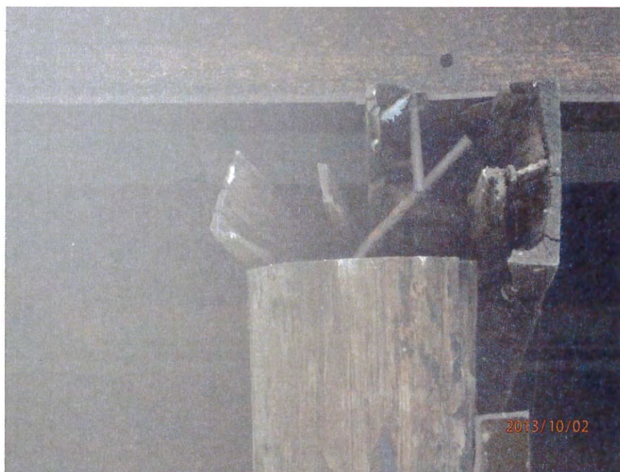
Photo 3-11 – Rotted and Crushed Timber Pile Cap
