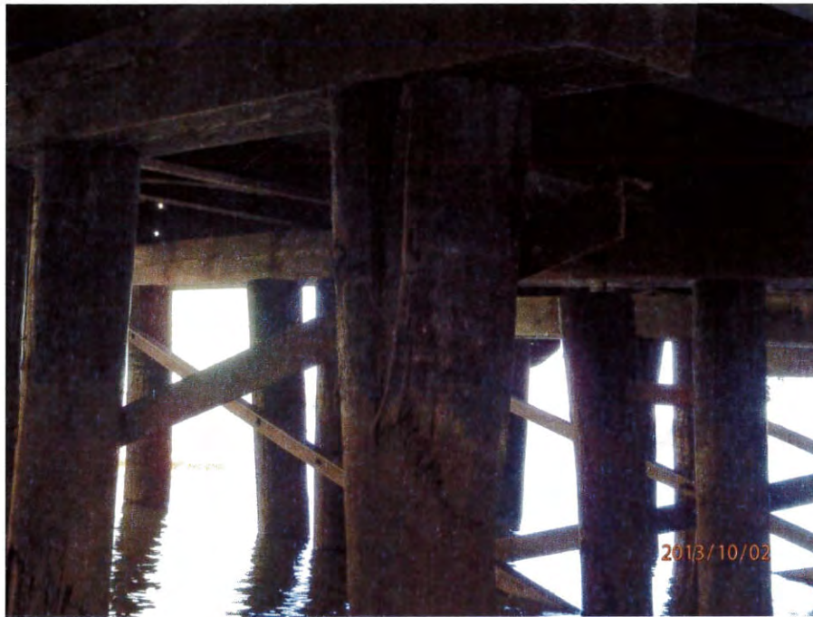
Photo 3-7 – Outboard Face of Pier, Adjacent Broken Piles
