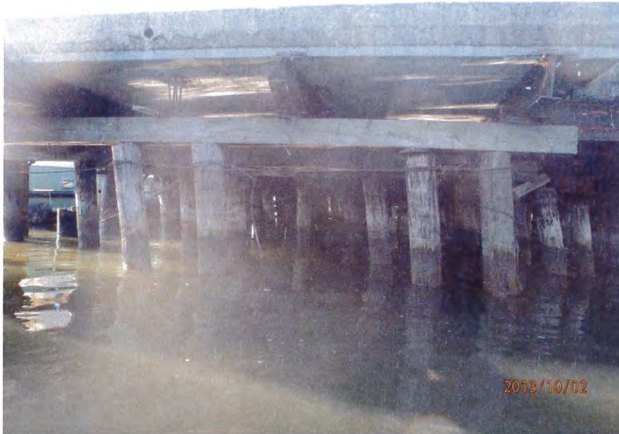
Photo 3-4 – Northern End of Pier, Piles Leaning and Shimmed
