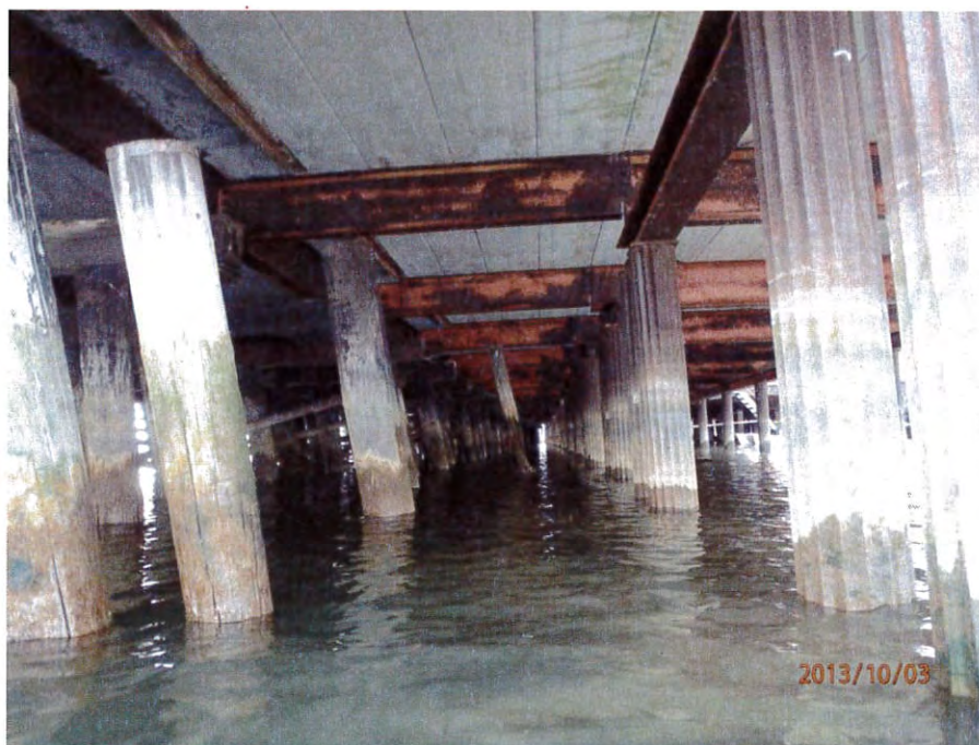
Photo 3-10 – Underside of Precast Panels in Good Condition
