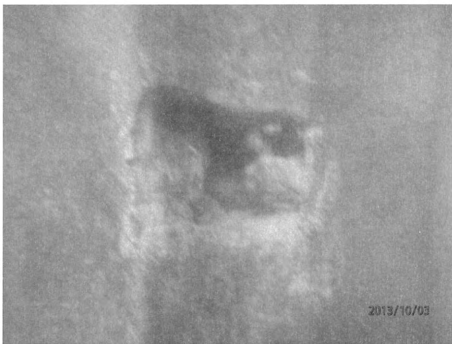
Photo 3-3 – Hole in Monotube, Concrete Fill Visible
