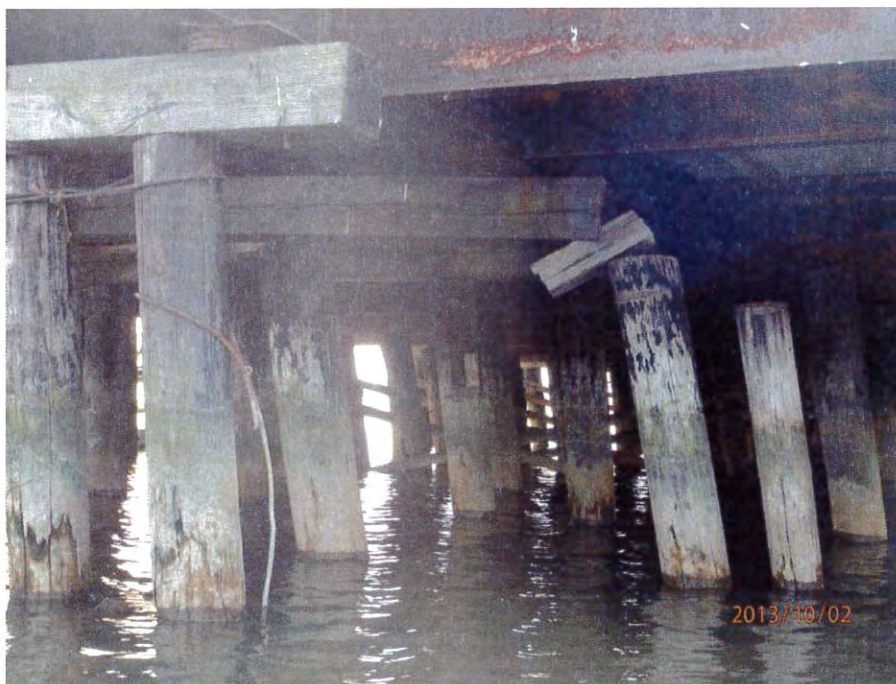
Photo 3-6 – Northern End of Pier, Limited Bearing on Cap
