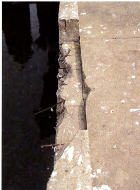
Photo 3-15 – Damaged Curb and Deck at North End, Precast Reinforcement Exposed
