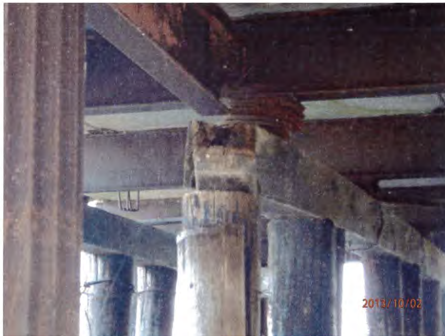
Photo 3-9 – Outboard Face of Pier, Shimmed Steel Framing
