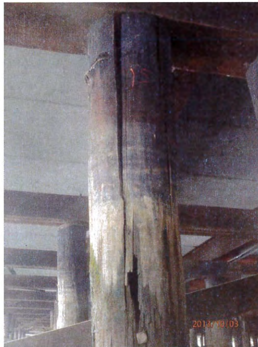
Photo 3-8 – Split and Hollow Timber Pile
