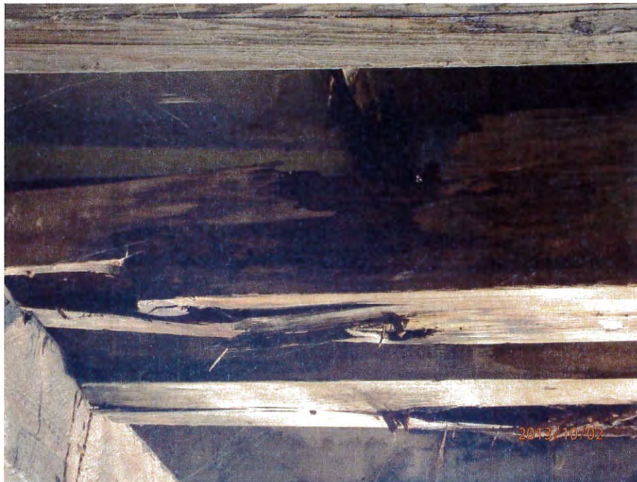
Photo 3-13 – Rotted and Failed Timber Joist at South End
