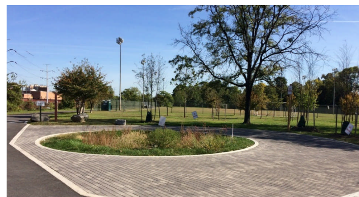
Permeable Pavers and Bioretention Cell, 4MR Park
