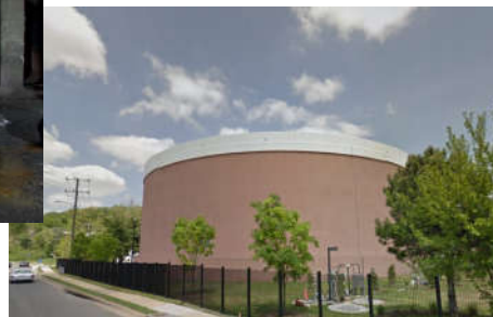
Arlington: Water Pollution Control Plant
