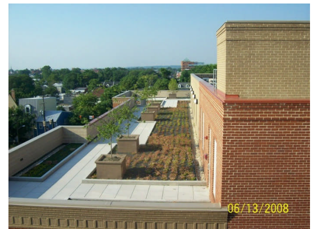
The Henry Green Roof
