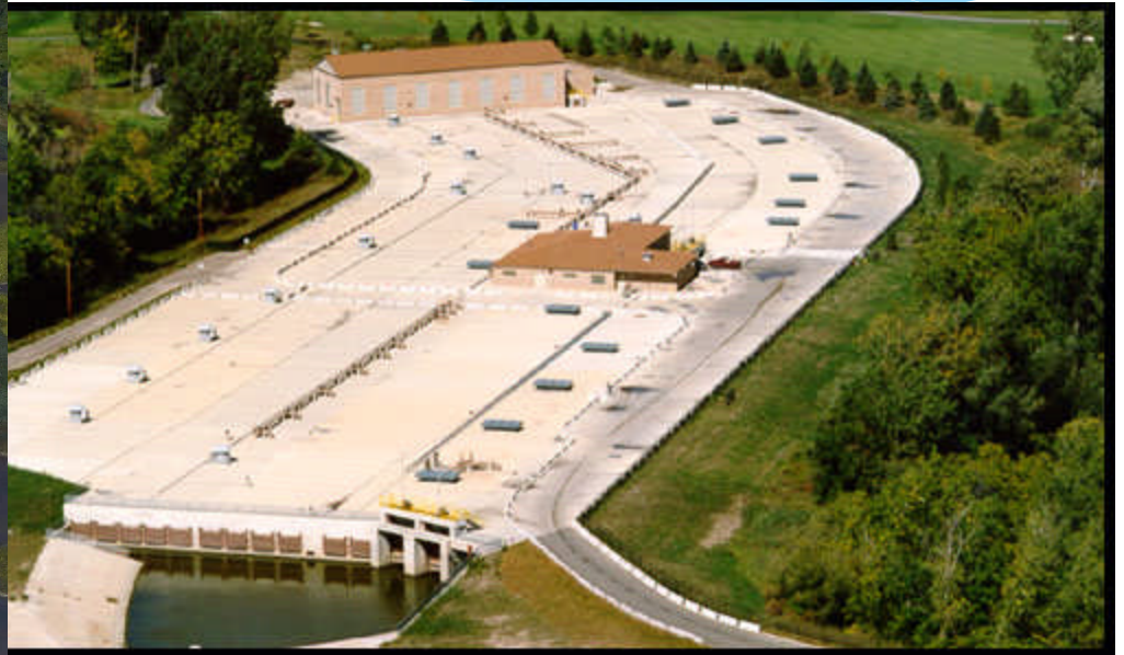
Detroit: Hubbell-Southfield CSO RTB
