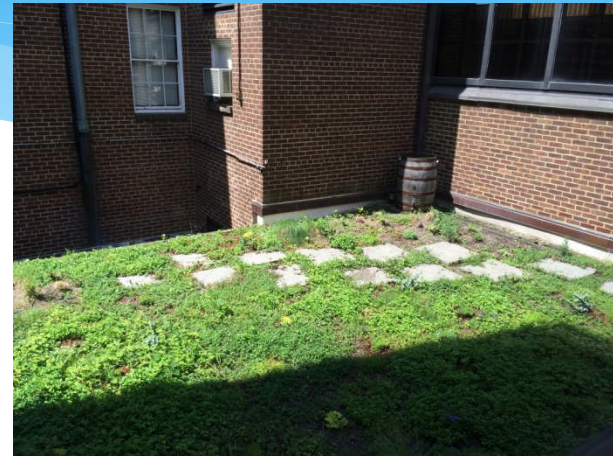
City Hall Green Roof
