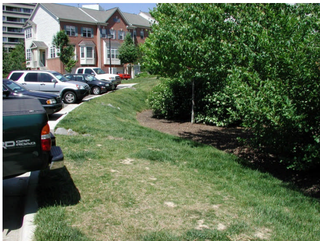
Kensington Court Bioretention
