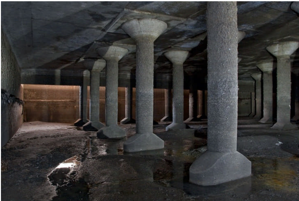
Toronto: Keelesdal-Hyde Ave Underground CSO Storage Tank
