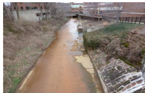
Prohibit CSOs during Dry Weather
