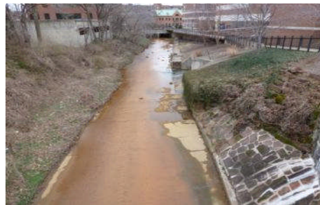
Prohibit CSOs during Dry Weather
