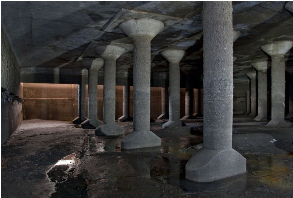
Toronto: Keelesdal-Hyde Ave Underground CSO Storage Tank
