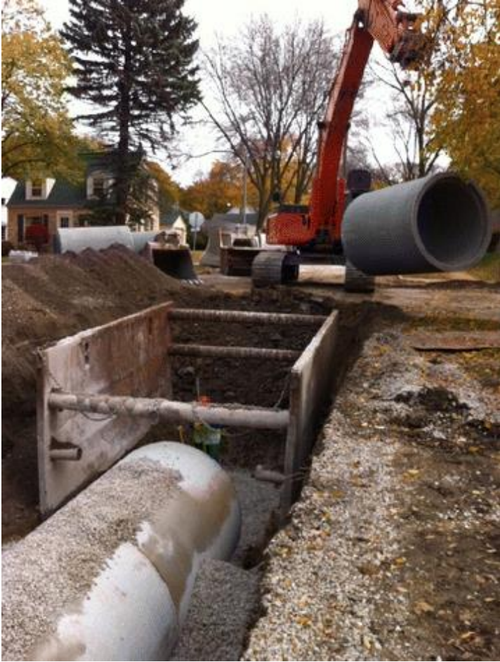
Hooffs Run Tunnel (open-cut)
