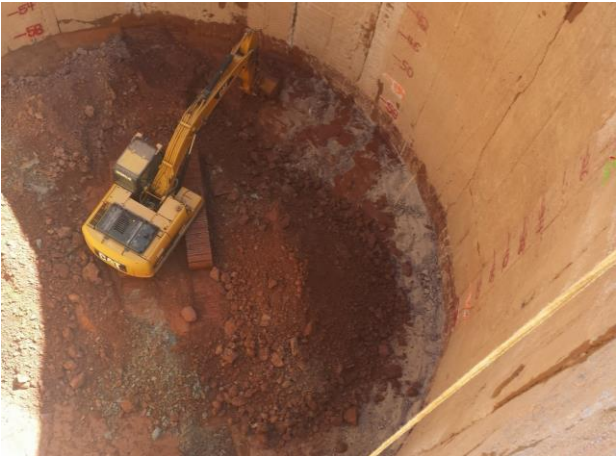
Shaft excavation
