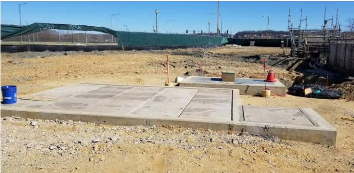
Shaft cover and backfill
