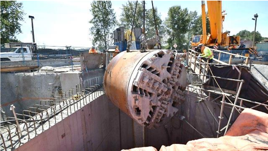
TBM removal
