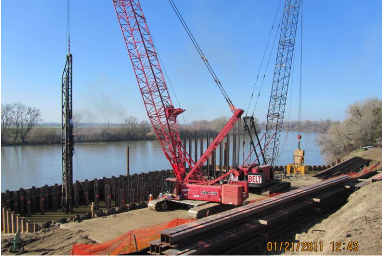
Work within sheet pile wall
