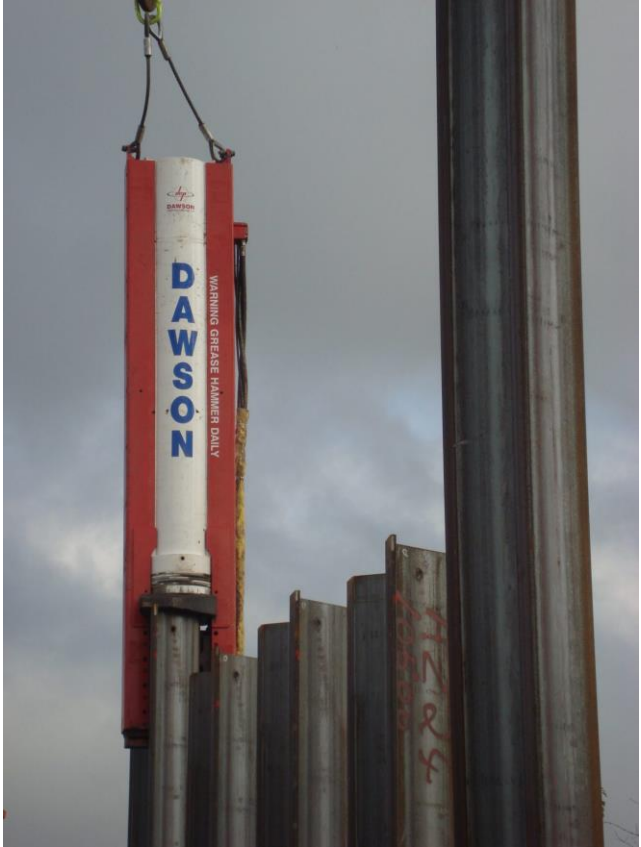
Sheet pile hammer
