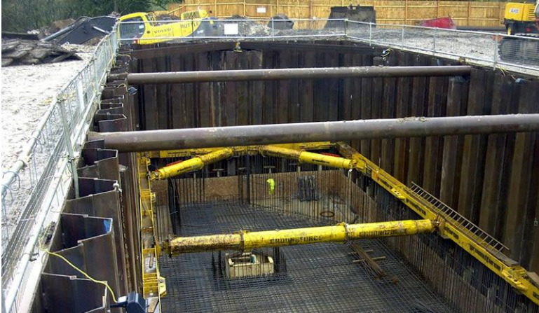
Braced sheet pile wall
