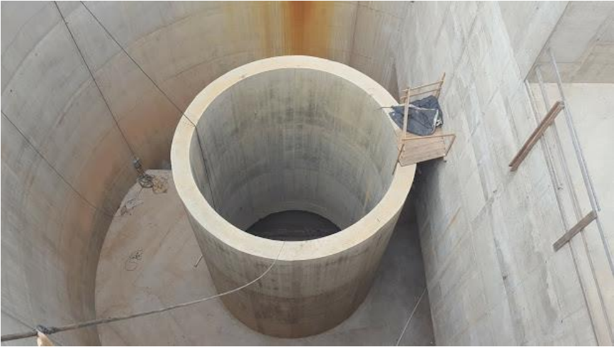
Shaft internal concrete (lower shaft)
