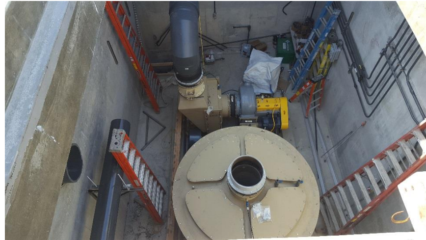
Equipment installation (where necessary)
