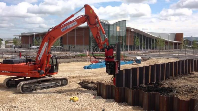
Sheet pile installation
