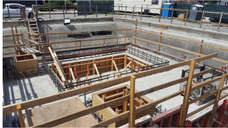
Concrete formwork and pours
