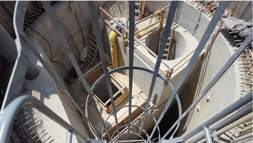
Shaft internal concrete (upper shaft)
