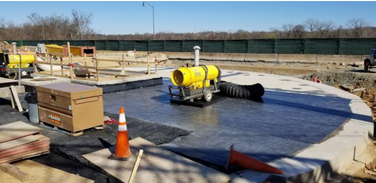
Shaft cover and backfill
