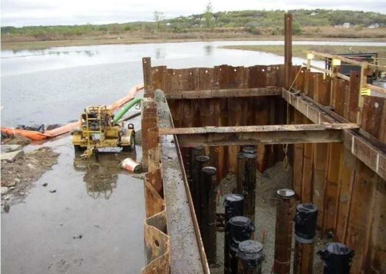
Finished sheet pile wall
