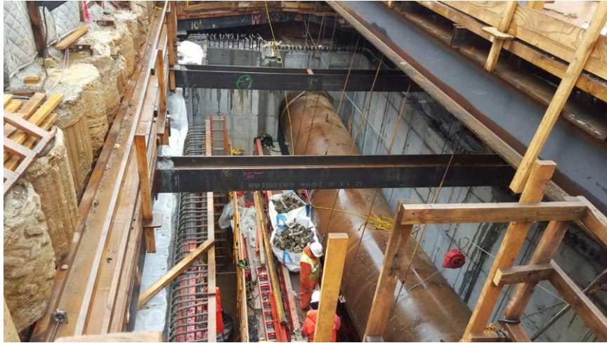
Excavation support and flume
