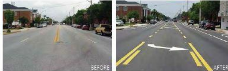
Before and after photos of a Road Diet project.
