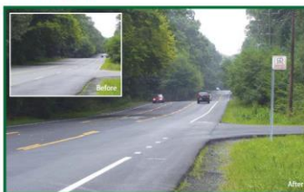
Lawyers Road, before and after a 2009 Road Diet Source: Randy Ottbemer, Virginia DOT
