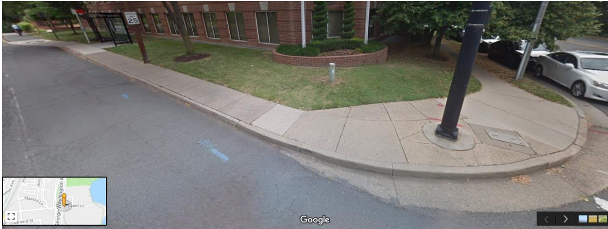
E Abingdon Drive, looking north. This current sidewalk will be widened into the existing bus pullout area, and the ramp will be upgraded.
