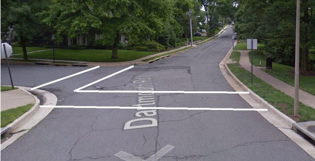
Dartmouth Road, looking east toward Princeton Boulevard. White bars show approximate proposed crosswalk location.
