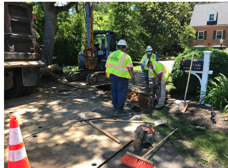
Rebuilt Public Storm Pipe on Janneys Lane
