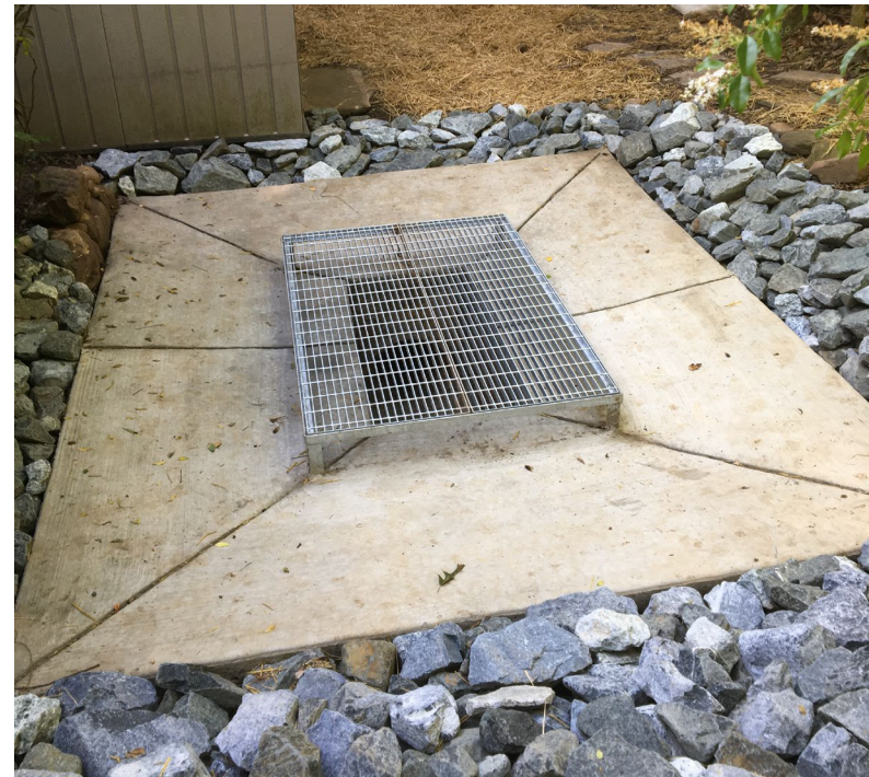
Rebuilt Structure on Ruffner Road
