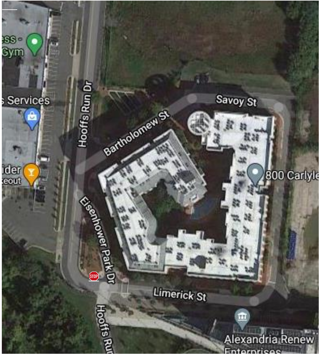
Aerial Image of Limerick Street at Hoofs Run Drive. Also depicts location of Alexandria Detention Center, AlexRenew, and Multifamily building 800 Carlyle.
