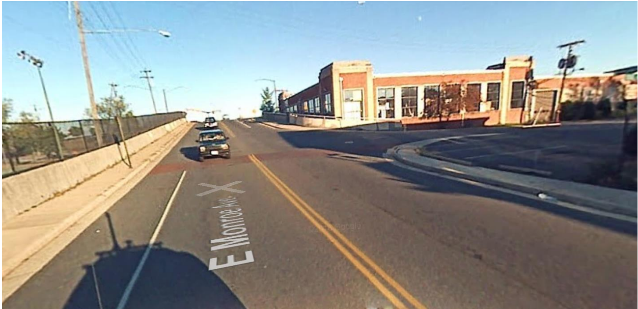
Monroe Avenue looking east towards Route 1 across the Leslie Avenue intersection
