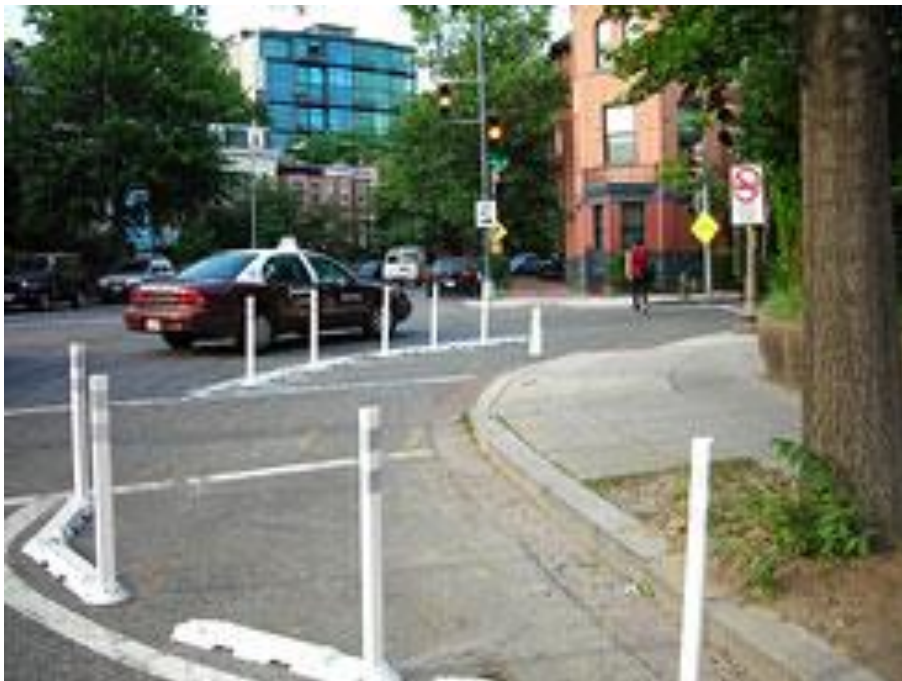
Bulbout with posts at 15 th and W Streets NW, Washington DC.
