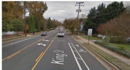
Buffered Bike Lanes King Street
