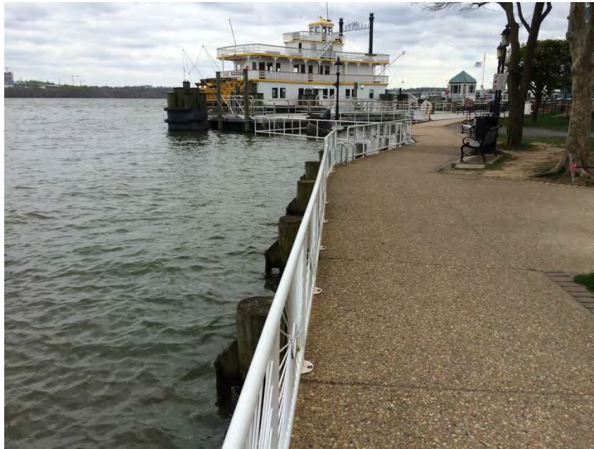
Photograph 3: Bulkhead along the waterfront at northern end of project, near the terminus of Thompson's Alley.
