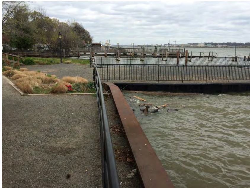
Photograph 6: Bulkhead along the waterfront at southern end of project, near the terminus of Duke Street.
