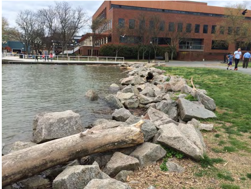
Photograph 1: Riprap stabilized shoreline at northern end of project, adjacent to Founders Park and near the terminus of Queen Street.
