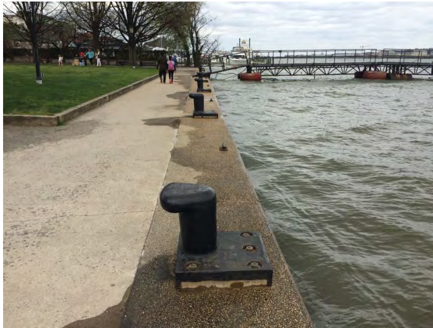
Photograph 5: Bulkhead along the waterfront at southern end of project, adjacent to Waterfront Park and near the terminus of Prince Street.
