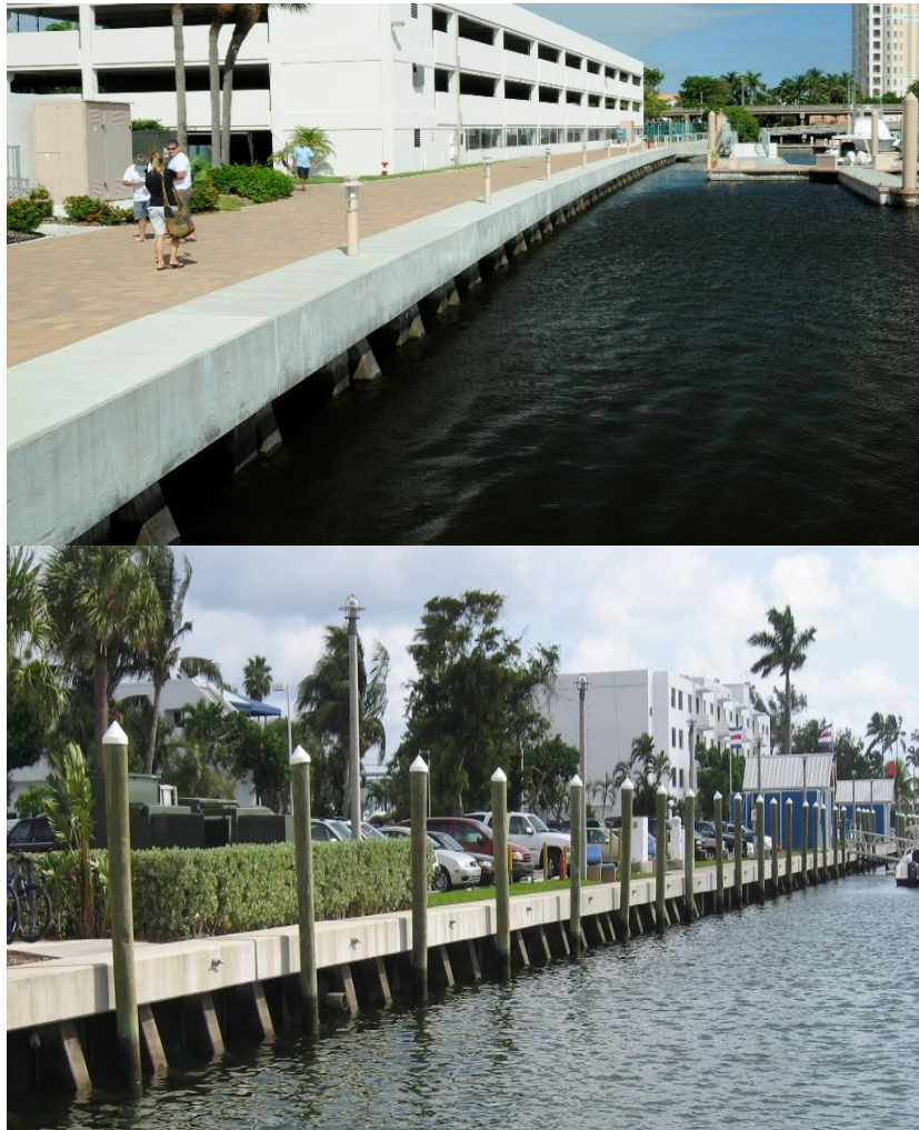
FIGURE 9: TYPICAL BATTER PILE BULKHEAD INSTALLATION
