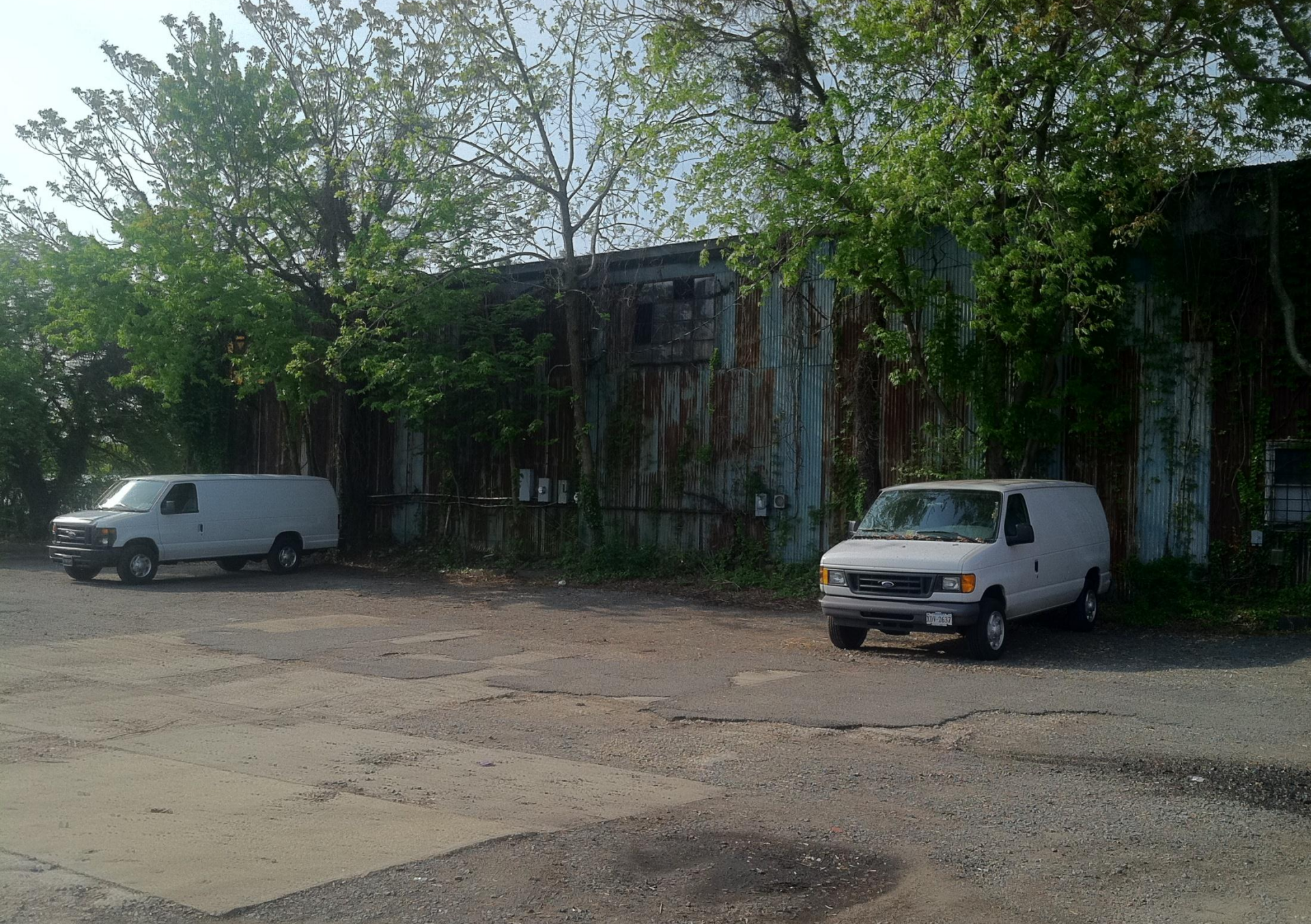
POINT LUMLEY PARK - EXISTING
