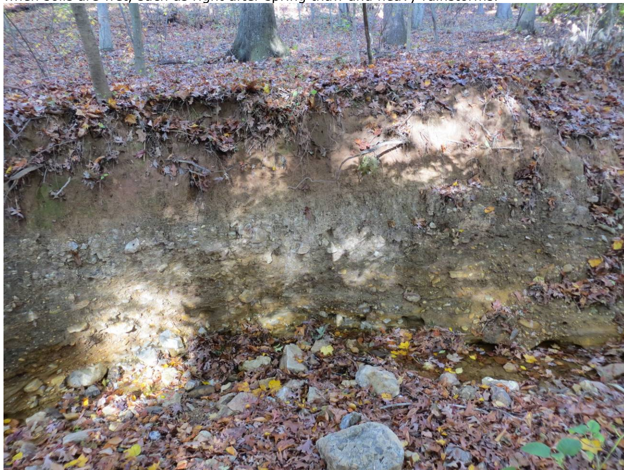
Figure 5-15. Crude slope-parallel stratification of weathered high-level colluvium, exposed in the head of a ravine in Dora Kelley Park. Photo by Tony Fleming.
