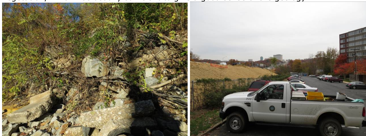
Figure 5-3. Examples of artificial fill. Left: heterogeneous fill composed of a mix of native soil, concrete fragments, and granite boulders not native to the City. Right: Shirley Highway rides on a massive berm of fill derived mainly from local geologic materials. The example on the left is readily recognizable as artificial fill because of its exotic components; the one on the right might not be if the material was seen out of context. Photos by Tony Fleming.
