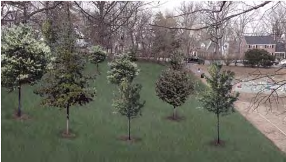
West Slope: Grassed/Natural Slope, 4H:1V slope
