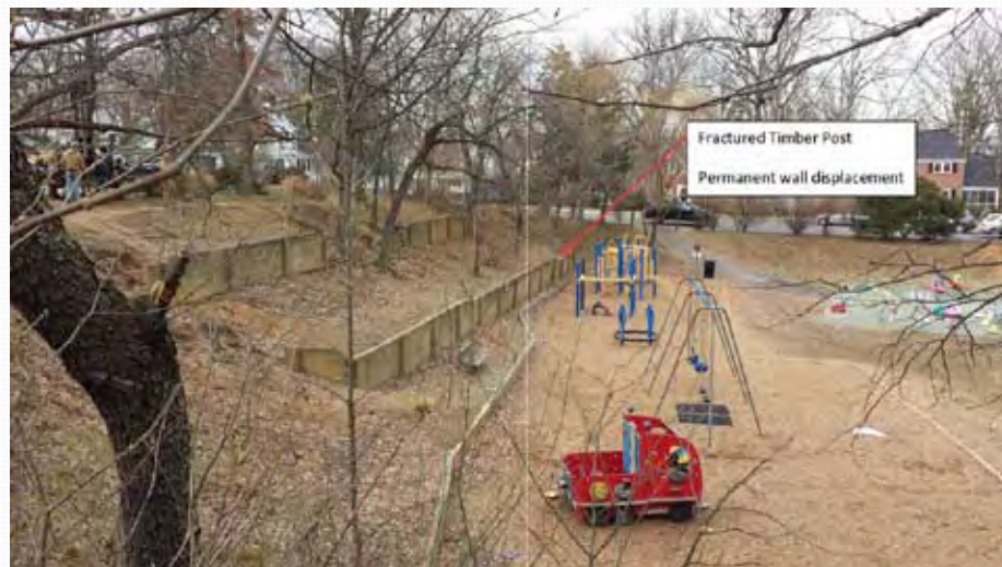
West Slope Retaining walls
