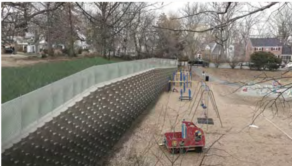
West Slope: 8.5' height retaining wall w/ 3' height handrail
