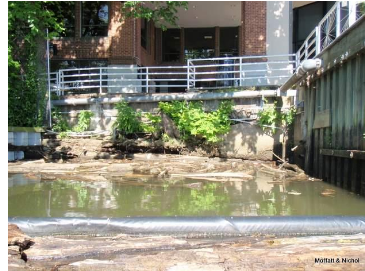
Figure 2-4: Debris Accumulation City Marina Ice
