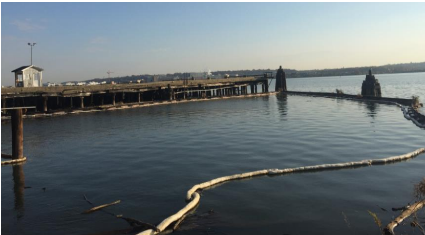
Figure 3-9: Existing RTN Facility
