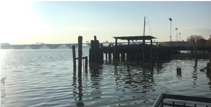
Figure 3-7: Existing RTS Facility
