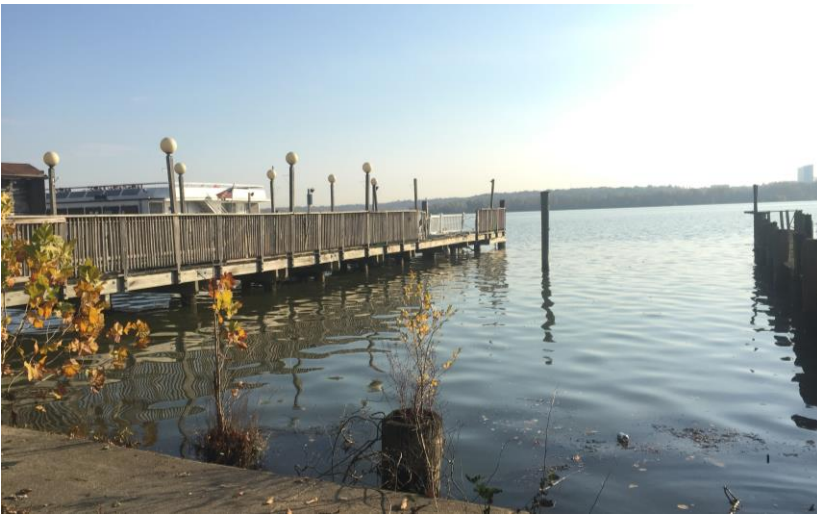
Figure 3-5: Existing Point Lumley Facility
