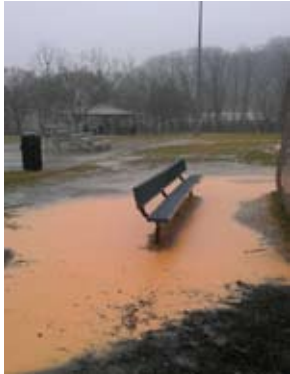
The current drainage issues at the ballfields cause the infield mix to wash off into the parking lot and surrounding areas after poor weather conditions.
