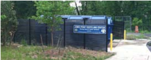
The City has a standard recycling drop-off center, as shown above in Jones Point Park.
