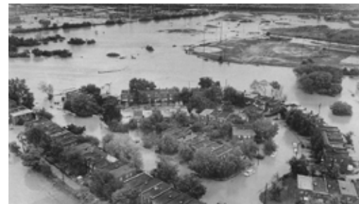
Flooding from Four Mile Run prior to channelization of the stream.
