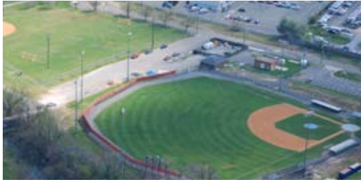
The Four Mile fields are amongst the best in the City, but need improved drainage systems. Field #2 faces the wrong orientation for meeting standards.
