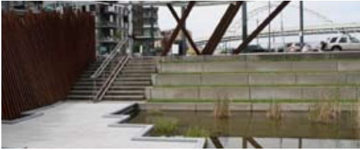
Integrated stormwater management in Portland, OR.
