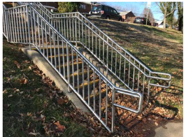
Handrail at stair
