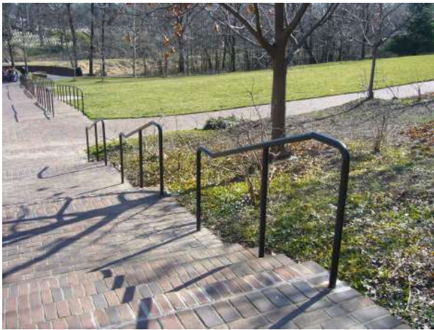
Handrail at stair
