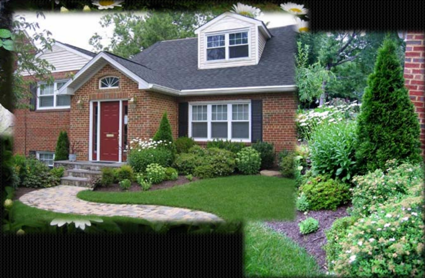
410 West Masonic View Avenue
