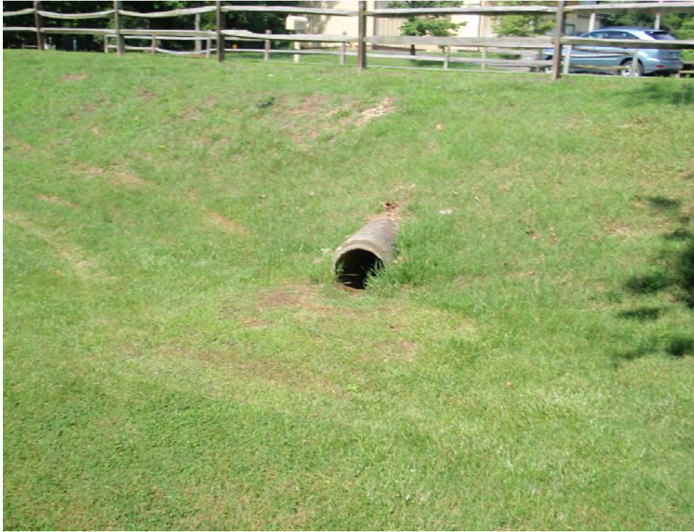
Figure B-4: Outlet of the 15-inch concrete pipe. No erosion was observed(Location ID #29)
