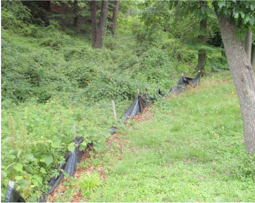
Figure B- 20: Silt fence downstream of the culvert (Location ID #43)
