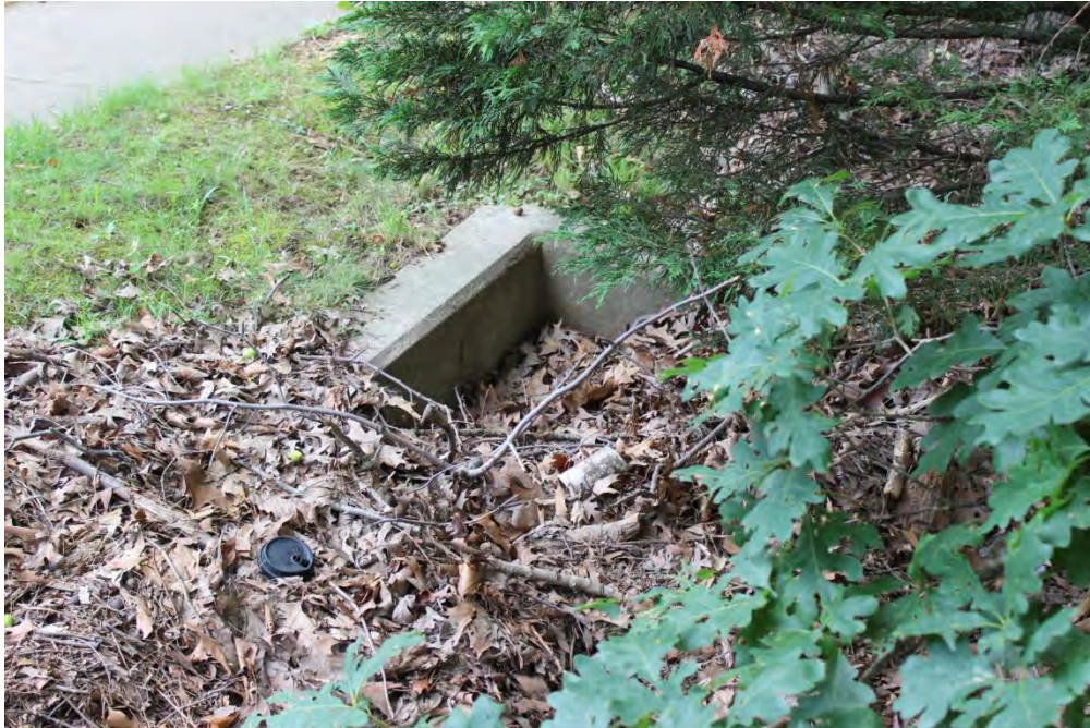
Figure B- 82: Inlet outfall at the Park property line (Location ID #109). Observed clogged inlet
