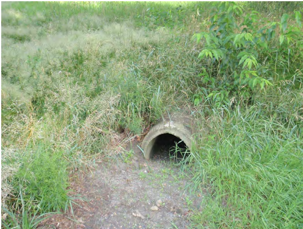
Figure B- 9: Outlet of 18-inch concrete pipe. Observed built-up debris and sedimentation, which may come from roadway (Location ID #30)
