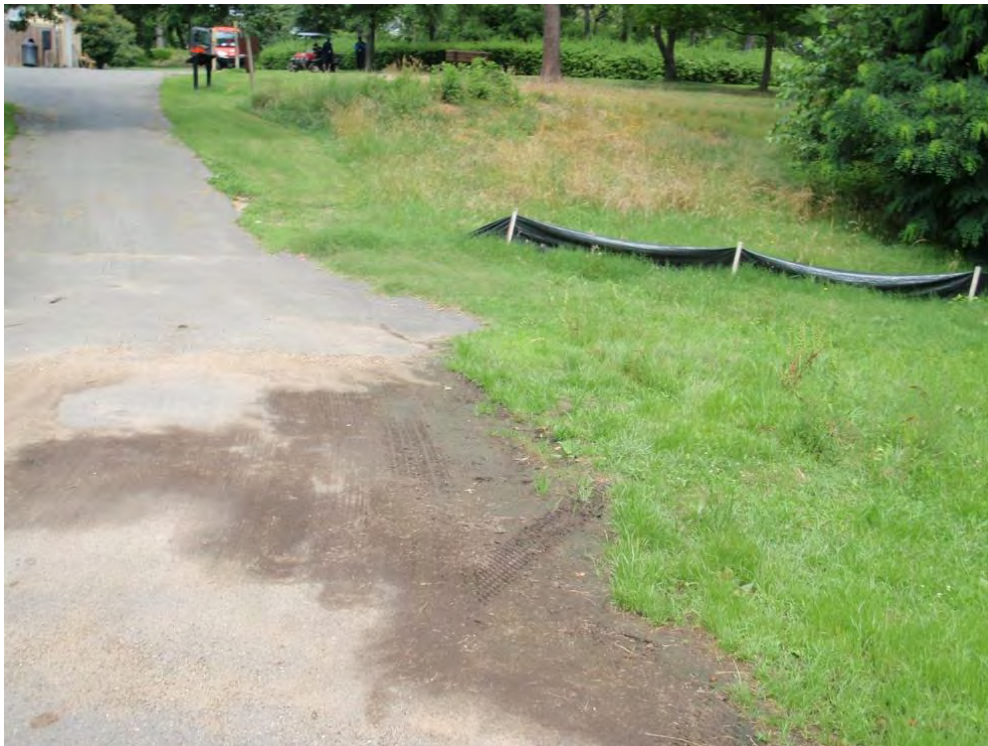
Figure B- 19: Road Crossing of the 36-inch culvert. Observed sedimentation at the road (Location ID #42)
