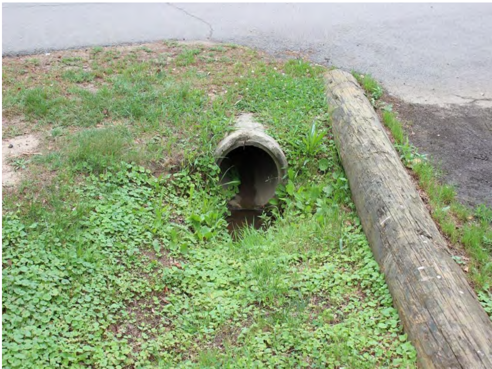
Figure B- 95: Inlet of the 15-inch culvert crossing (Location ID #122). Observed depression at the inlet
