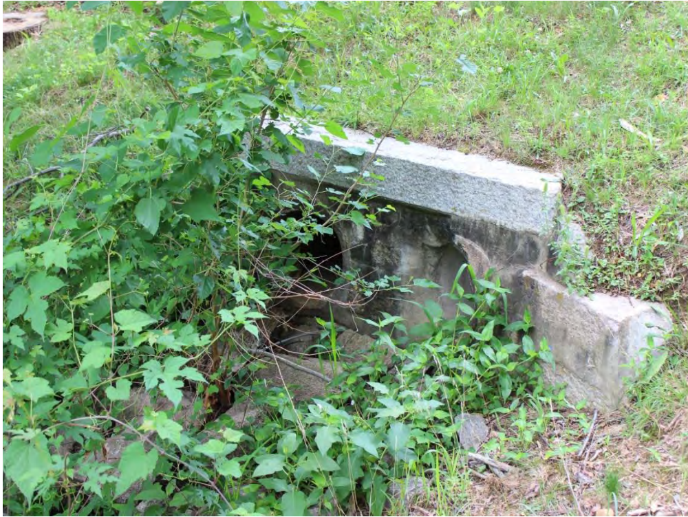
Figure B- 94: Outlet of the 15-inch culvert crossing (Location ID #121).
