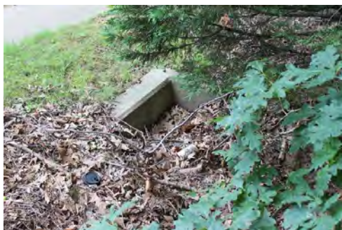
Clogged Inlet Outfall at the Park Property Line
