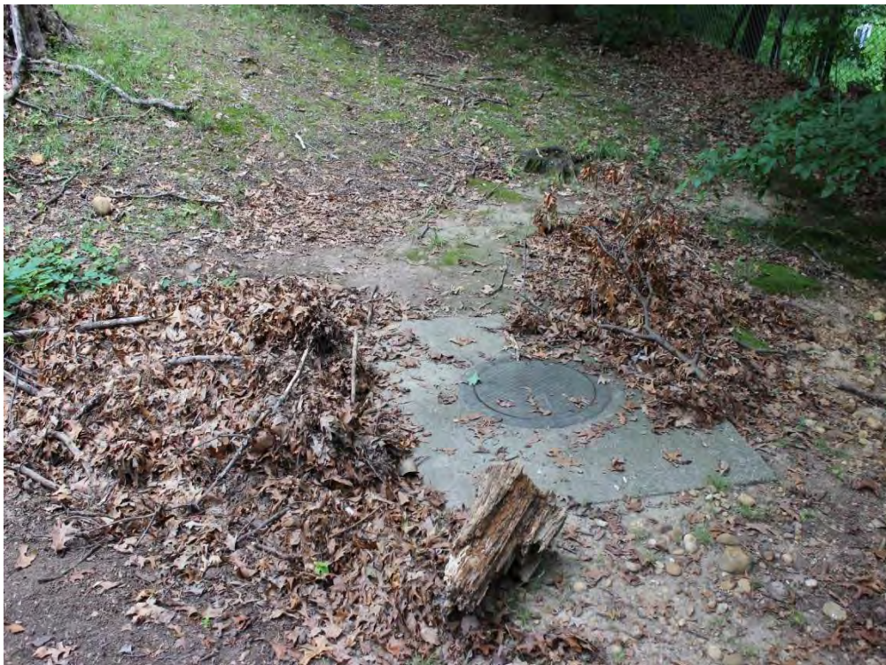
Figure B- 85: Inlet (Location ID #112). Observed built-up debris clogging the inlet
