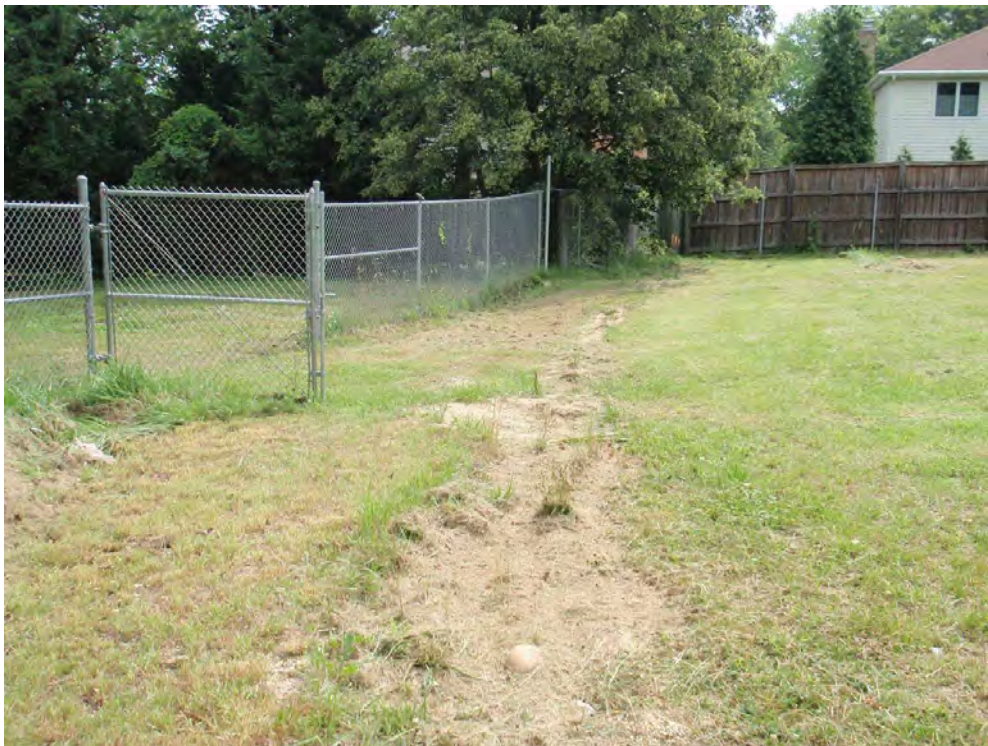
Figure B- 23: Trench drain along the chain-linked fence on the City property (Location ID #46)
