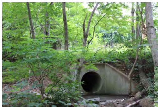
Inlet feeding into SWM pond from Marlboro Properties
