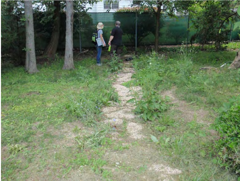
Figure B- 36: Trench drain. Homeowners covered the bare soil with mulch which helped to improve the drainage. Observed dry ground after the storm (Location ID #59)
