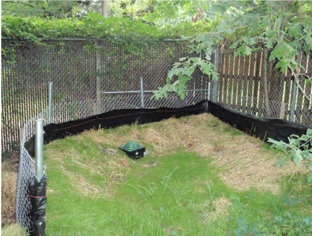
Figure B- 28: Catch basin as interim drainage solution (Location ID #51)
