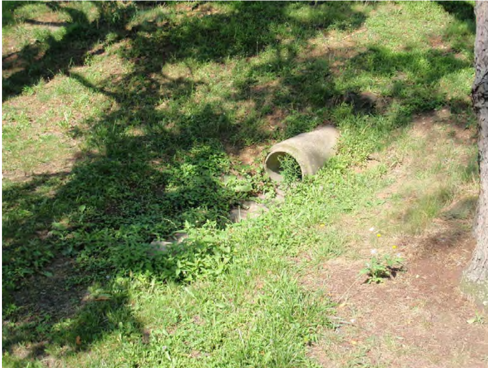
Figure B- 8: Outlet of the 15-inch concrete pipe (Location ID #28)
