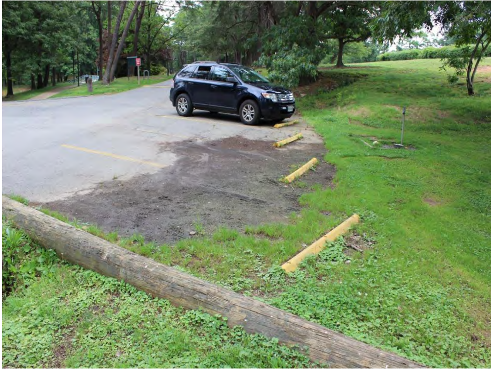
Figure B- 96: Parking lot next to the Inlet (Location ID #126). Observed sedimentation at the parking lot
