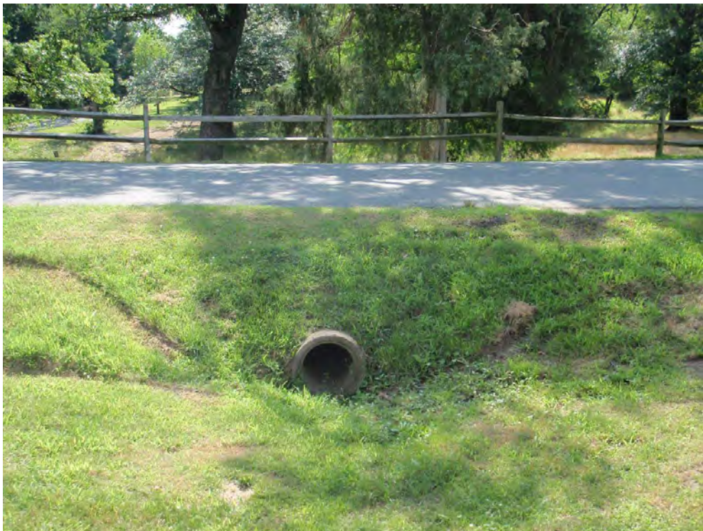
Figure B- 5: Inlet of the 15-inch concrete pipe next to the parking lot (Location ID #25). Observed a small ponding area at the inlet
