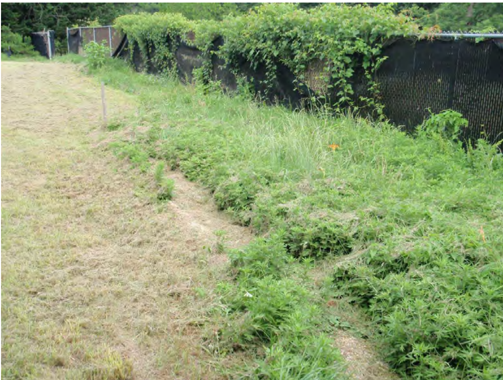
Figure B- 33: Trench drain along the fence (Location ID #56)
