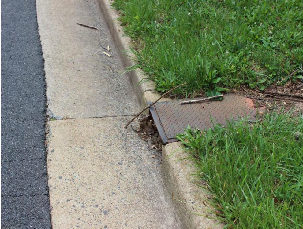
Figure B- 76: Outfall from the Park along N. Van Dorn Street (Location ID #103). Observed outlet clogged by debris
