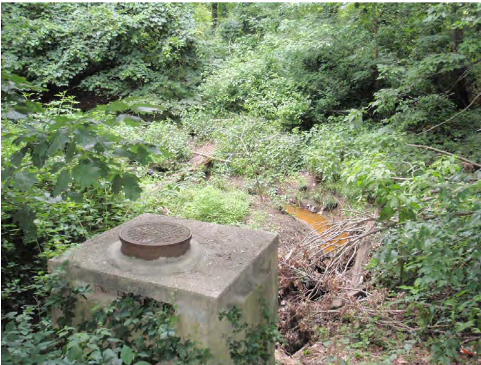
Figure B- 73: Stormwater management (SWM) pond riser (Location ID #100)
