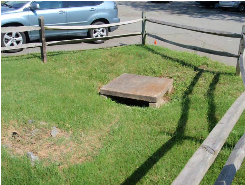
Figure B-2: Shallow drop inlet next to the parking lot (Location ID #23)
