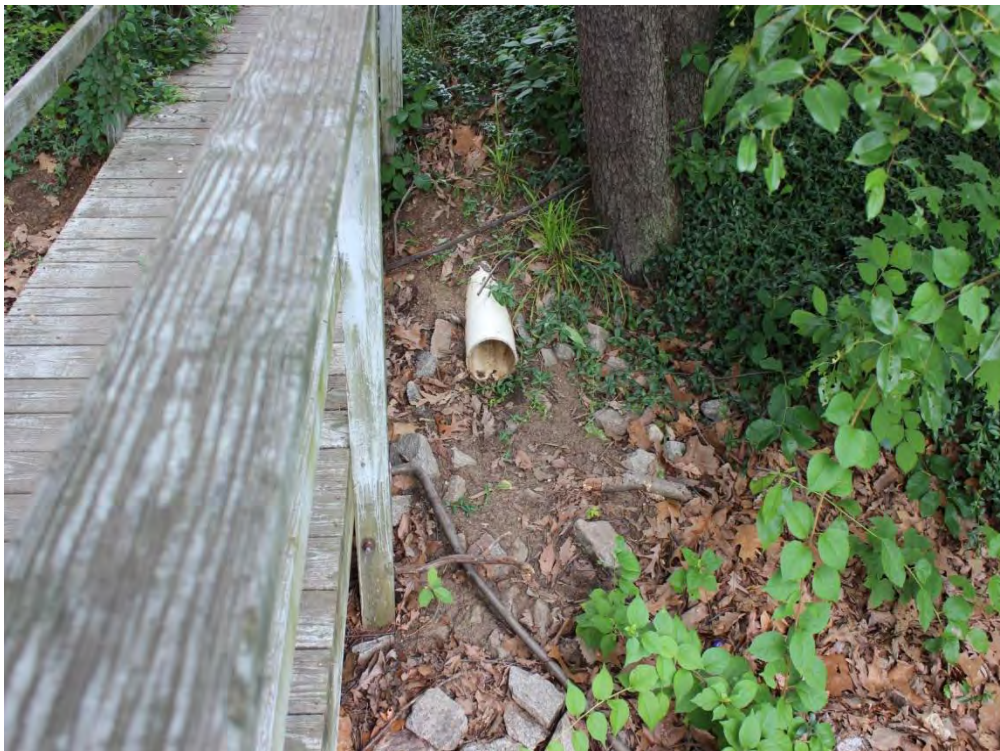
Figure B- 105: PVC Outlet by the footbridge. Observed clogging during previous storm events (Location ID #132)
