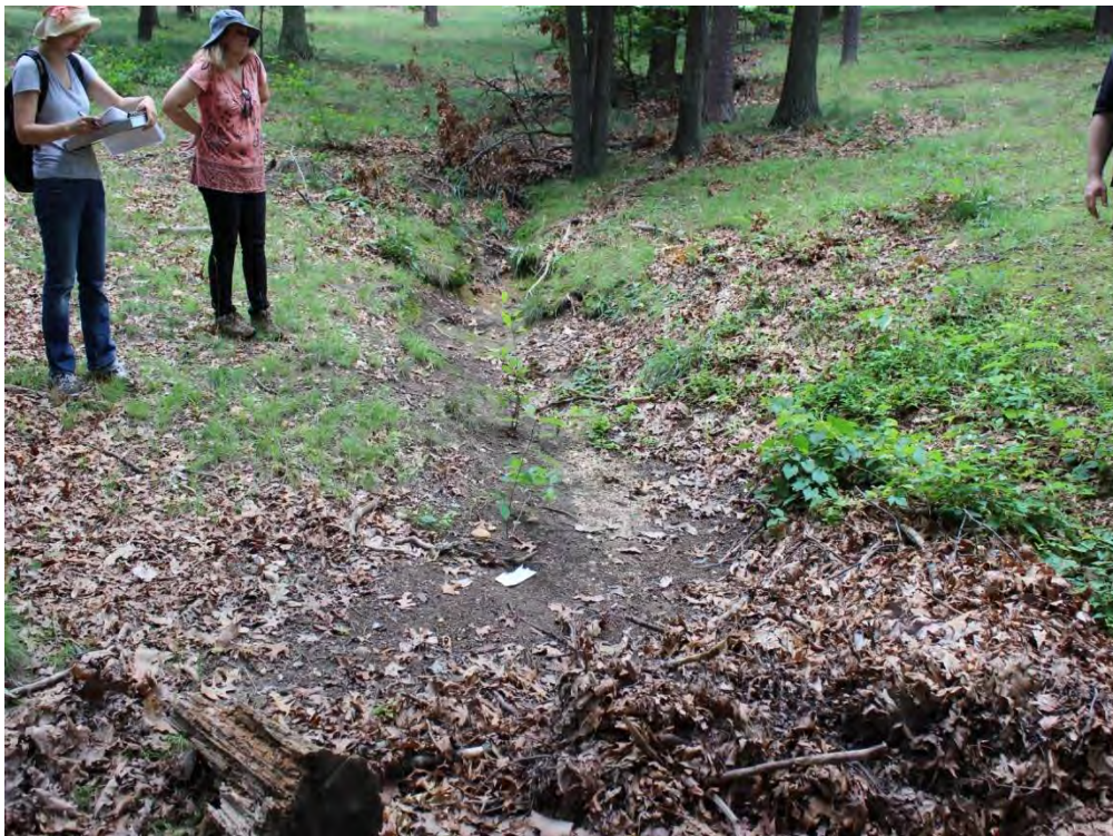
Figure B- 87: Upstream area of the inlet (Location ID #114). Observed debris and sedimentation
