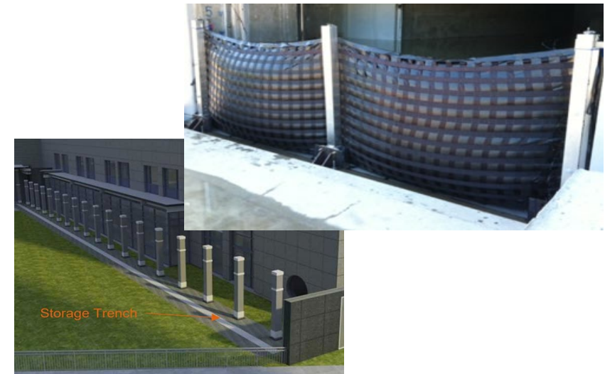
Concealed on-site storage and flexible membrane flood barrier across building flood pathways
