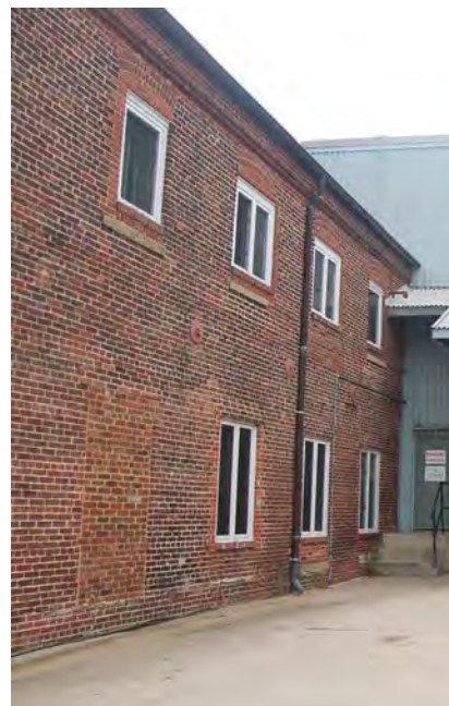
Figure 23. This detail of the circa-1864 photo of the coopers shop’s west elevation (on left) shows that the 2 nd -story windows were as large as the first story and had a straight header. The 2014 photo of 2 Duke Street’s west elevation (on right) shows that, although altered from the 1896 window conformation, the 2 nd -story windows were smaller and had a rounded jack arch header. (1864 photographer unknown; History Matters, LLC 2014)
