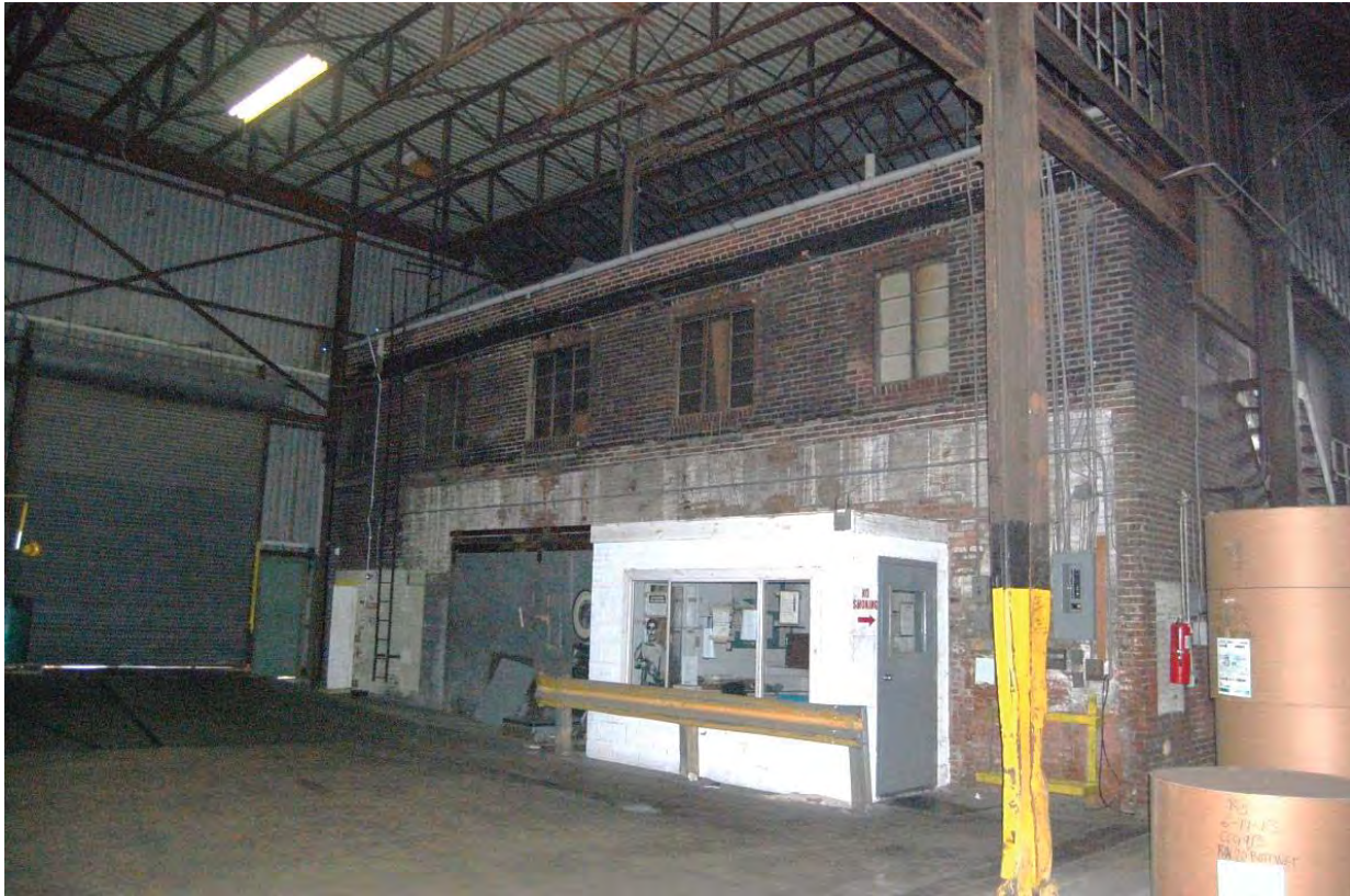
Figure 40. West elevation of 2 Duke Street on the south end. This photograph shows where Moore's 1896 blacksmith shop addition was attached to the building (white paint on the building). RTWC took over the building's operation in 1957, removed the addition, and added the small vestibule (painted white). (History Matters, LLC; December 2013)
