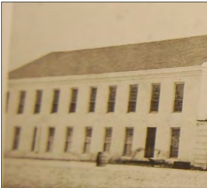
Figure 23. This detail of the circa-1864 photo of the coopers shop’s west elevation (on left) shows that the 2 nd -story windows were as large as the first story and had a straight header. The 2014 photo of 2 Duke Street’s west elevation (on right) shows that, although altered from the 1896 window conformation, the 2 nd -story windows were smaller and had a rounded jack arch header. (1864 photographer unknown; History Matters, LLC 2014)
