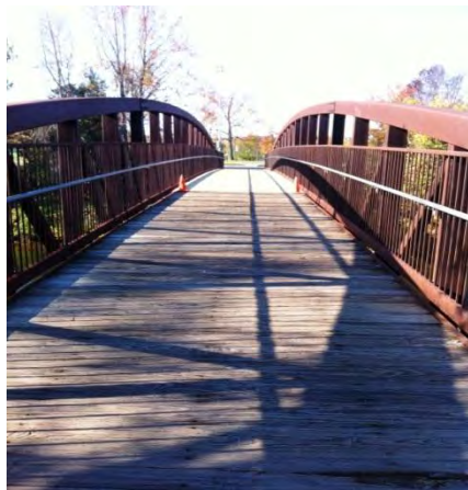
Before (with old decking)
