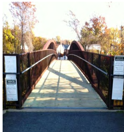
After (with new decking)
