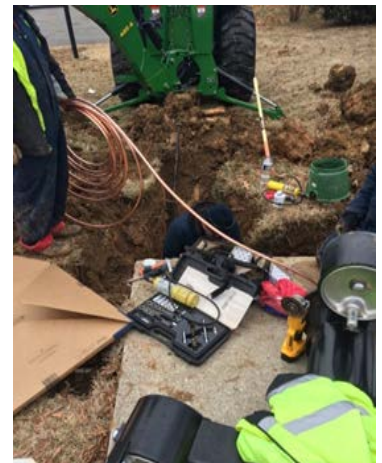
Valve replacement for irrigation
