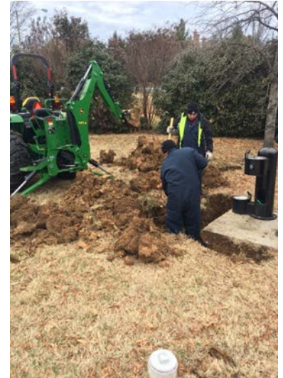
Valve replacement by staff for irrigation
