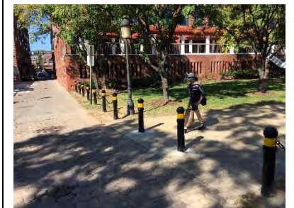
City Standard Bollards- Thompson's Alley
