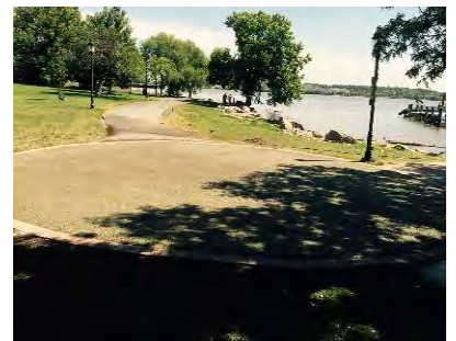
Porous Pave Installation
