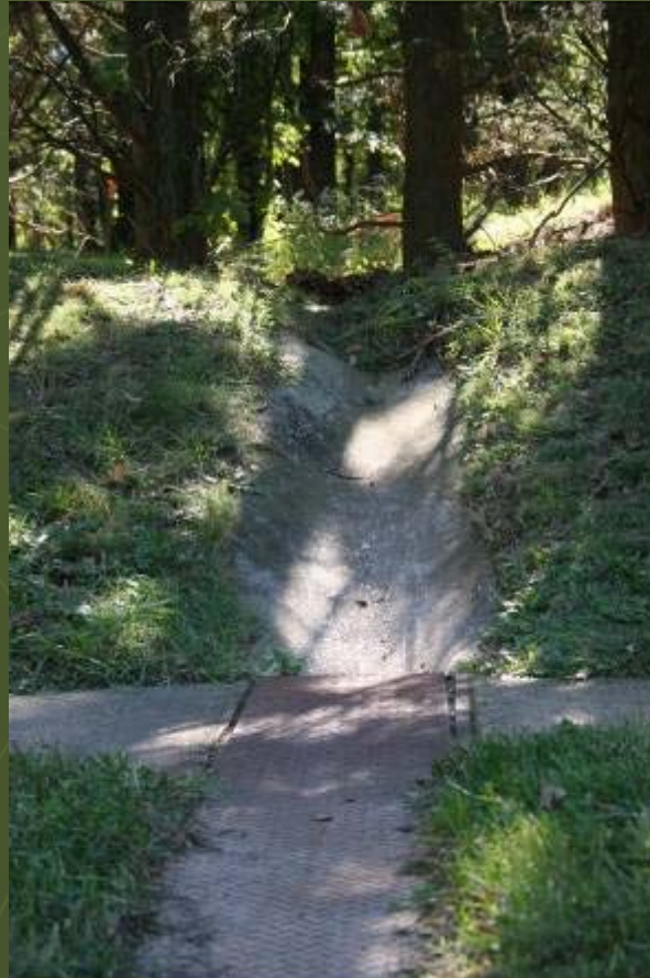
Trough From Park Under Sidewalk @ Van Dorn St.
