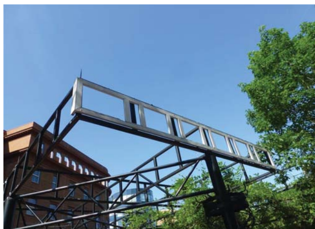
Figure 62. A secondary wood trellis, painted white, has been attached to the major trellis system; the purpose is unknown.
