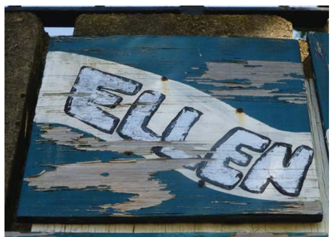
Figure 29. Corrosion of ferrous screws has led to staining and failure of the fasteners, typical.
