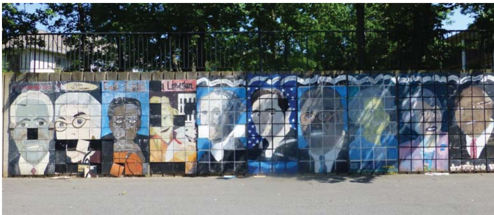
Figure 24. The community project mural exhibits advanced deterioration due to extensive failure of the plywood.
