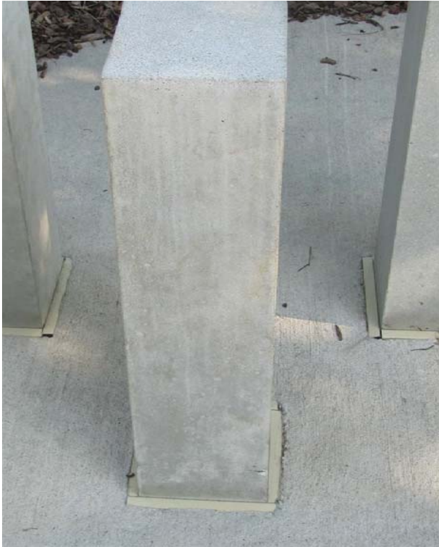
Figure 15. Detail of typical water run-off/streaking pattern down the face of one of the pillars.
