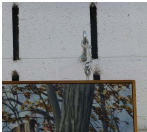
Figure 116: Detail of the mounting hardware used to affix the panels to the wall.
