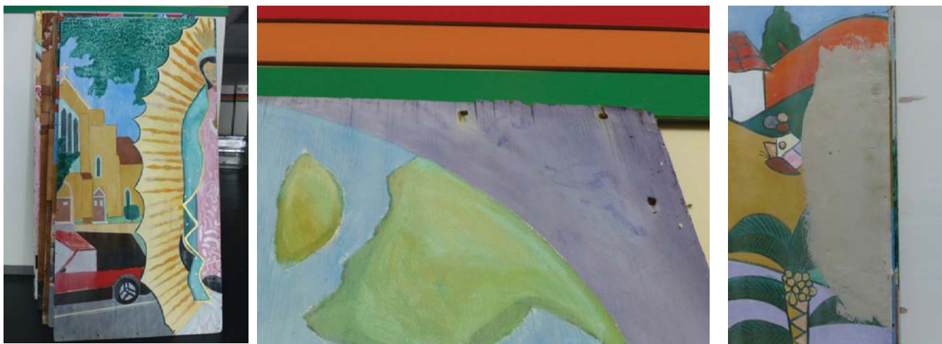
Figure 79 (left). Each panel measures approximately 4'x8'. Figure 80 (center): The edges of each board are warped and frayed. Figure 81 (right): An area of rot has been cut out and new wood spliced in.
