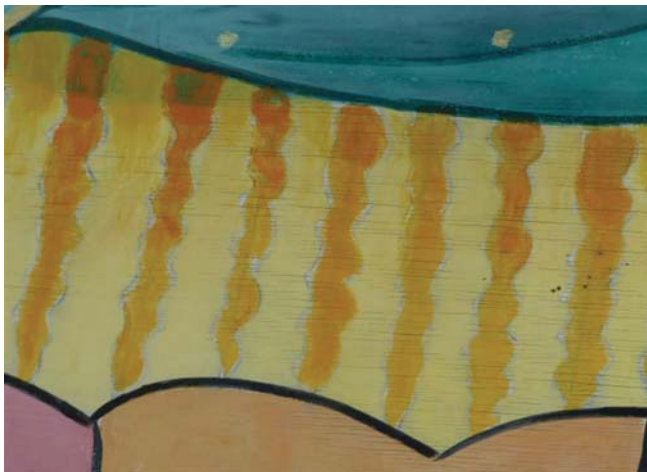
Figure 82. Shrinkage and warping of the plywood panel has led to cracking of the surface paint.
