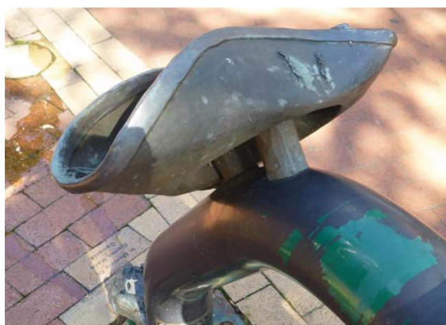
Figure 64. The steel and bronze water fountain exhibits surface deterioration including loss of protective coatings and corrosion.
