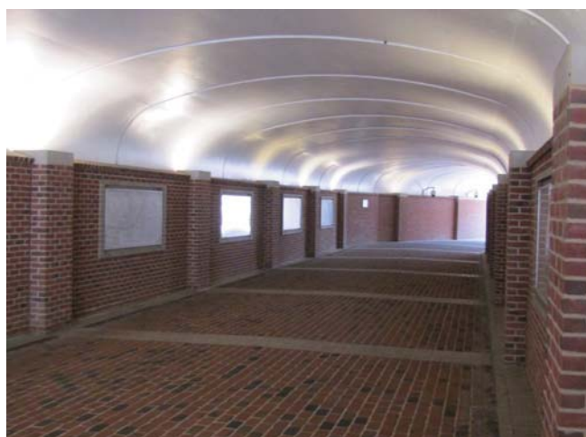
Figure 48. General view of the concourse setting.
