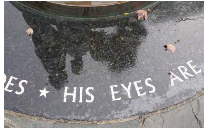
(Left) Figure 3. Slate pavers exhibit minor flaking and mortar loss typical to a highly-trafficked surface. (Right) Figure 4. Paint is flaking from within the lettering on the inscribed granite pavers.
