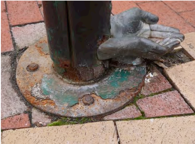
(Left) Figure 11. Detail of advanced corrosion on the steel base of the water fountain with bronze sculptural features.
