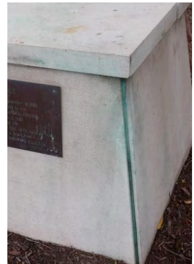
(Left to Right): Figure 1. Brio measures 8' in height including plinth. Figure 2. The cast stones of the pedestal have become displaced. Figure 3. Copper staining has discoloured the joints.
