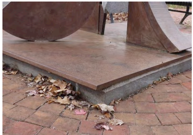
Figure 4. Iron staining of the granite base and vegetative growth in the pavers abutting the sculpture.
