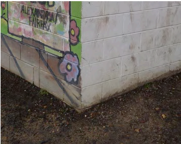
(Left) Figure 7. Splash- back from the ground below has soiled the lowermost 12" of the mural.
