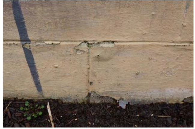
(Left) Figure 1. Overall view of the mural on the north side of the building. (Right) Figure 2. Detail of one of the instances of paint blistering and loss.
