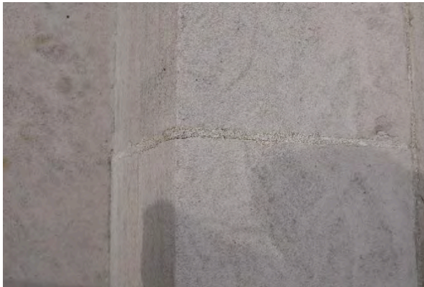
Figure 5. Detail of typical caulk joint at base.
