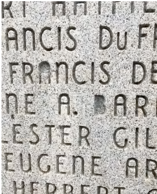
Figure 3. Small stone stubs from within "A"s and "B"s have begun to spall off.
