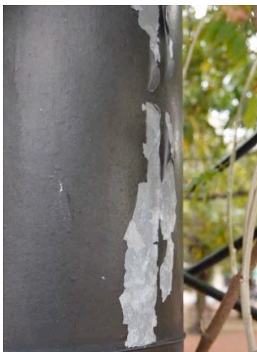
(Left) Figure 3. Detail of paint loss on a steel structural member revealing the galvanized surface below.
