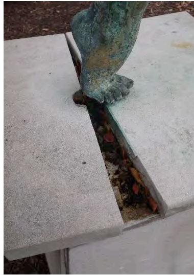
(Left to Right): Figure 1. Brio measures 8' in height including plinth. Figure 2. The cast stones of the pedestal have become displaced. Figure 3. Copper staining has discoloured the joints.
