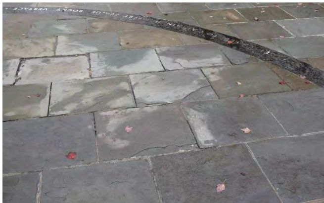
(Left) Figure 3. Slate pavers exhibit minor flaking and mortar loss typical to a highly-trafficked surface. (Right) Figure 4. Paint is flaking from within the lettering on the inscribed granite pavers.
