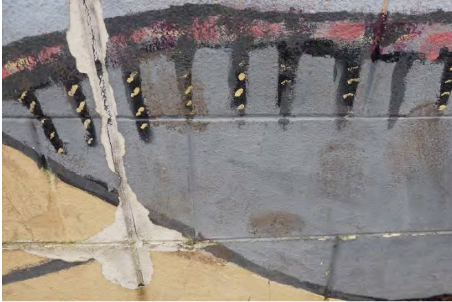
(Left) Figure 5. Flaking of the topcoat reveals the primer underneath.
