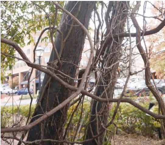
Figure 7. Vegetation on steel introduces water to the metal surface.
