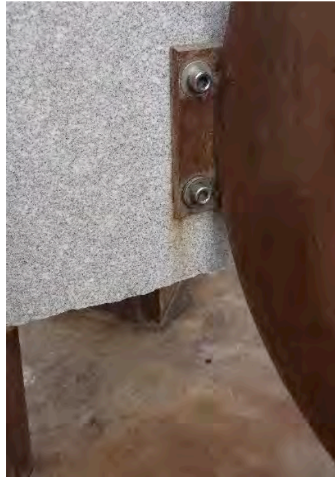
Figure 2. Detail of iron staining the granite.
