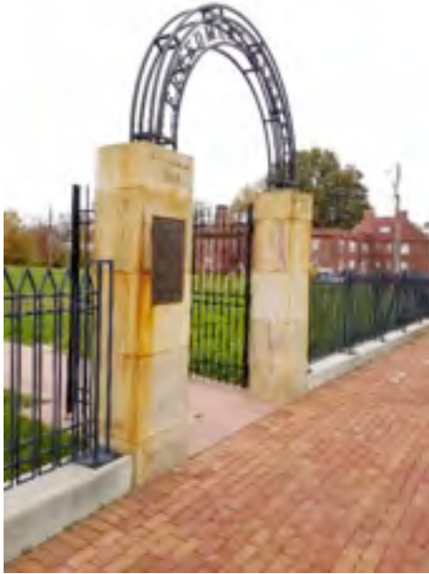
(Left) Figure 5. Cemetery entrance; the sandstone pier shows severe iron-staining from the ferrous bolts. (Right) Figure 6. View of the north wall (interior facing) with bronze plaques.
