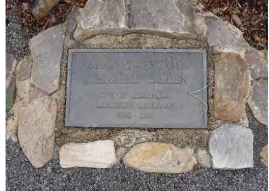
Figure 2. Detail of general soiling and deterioration of plaque.
