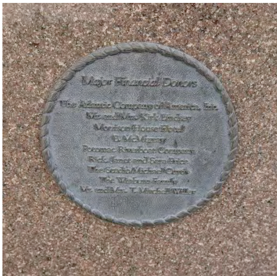
(Left) Figure 4. Two of the three circular plaques have little to no wax coating remaining and are corroded.
