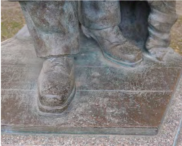
(Left) Figure 6. Minor pitting on edges of figure's shoes, may be an original casting flaw.
