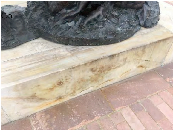
(Left) Figure 3. Sandstone wall exhibits iron and copper staining.
