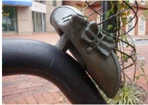
Figure 6. The steel and bronze water fountain exhibits surface deterioration including loss of protective coatings and corrosion.
