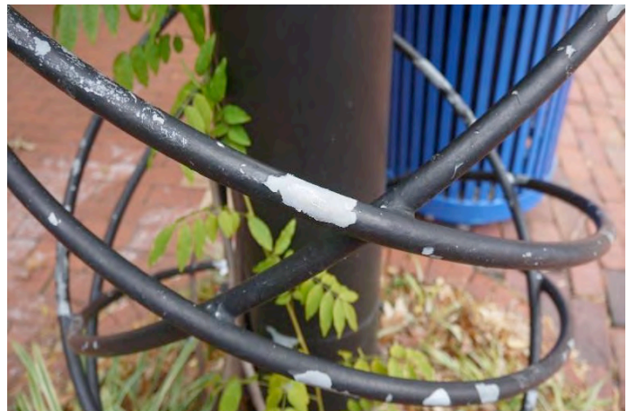
Figure 8. Detail of typical paint loss.
