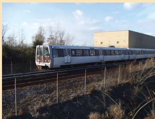
Existing Metrorail Blue/Yellow Line between Potomac Greens and Potomac Yard
