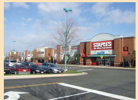
Existing Potomac Yard Shopping Center
