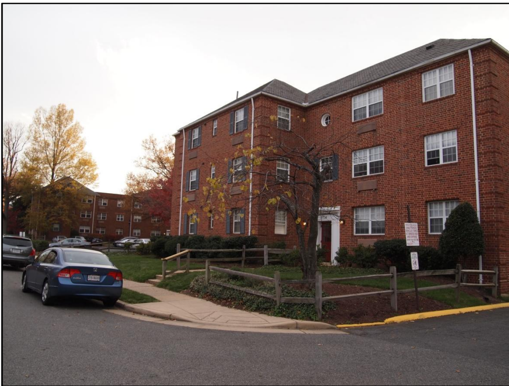
Plate 6: Abingdon Apartments, east elevation of a U-shaped building, view southwest.
