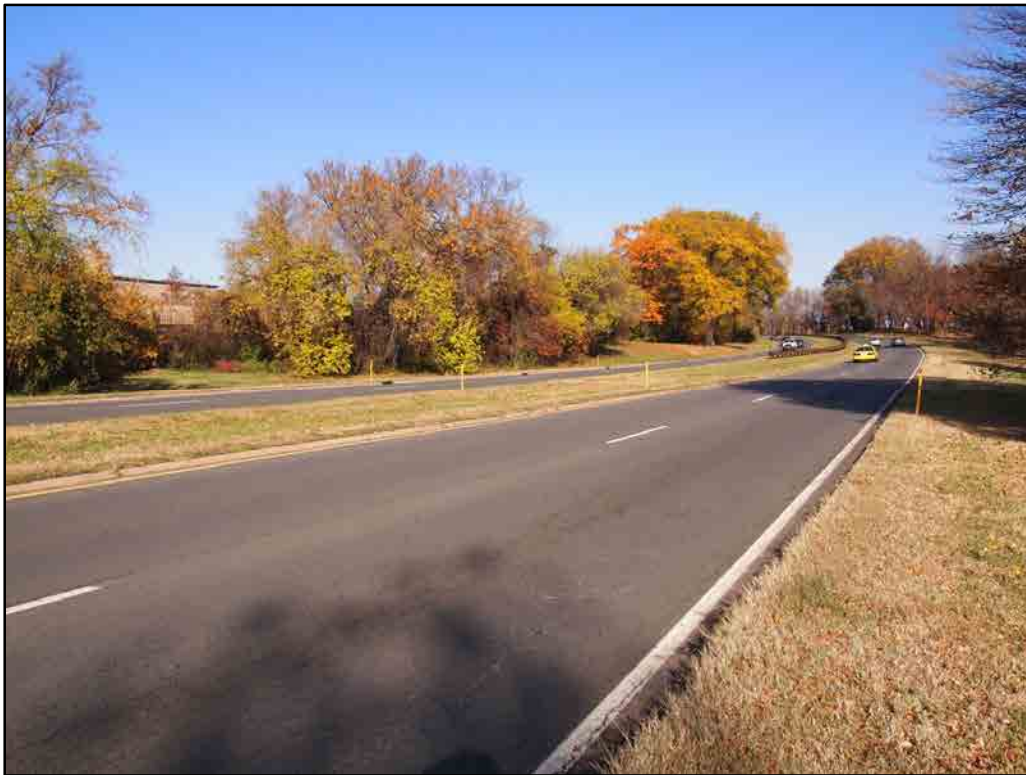
Plate 2: View north on the MVMH/PNCR east of the Regal Cinemas at Potomac Yard Shopping Center.
