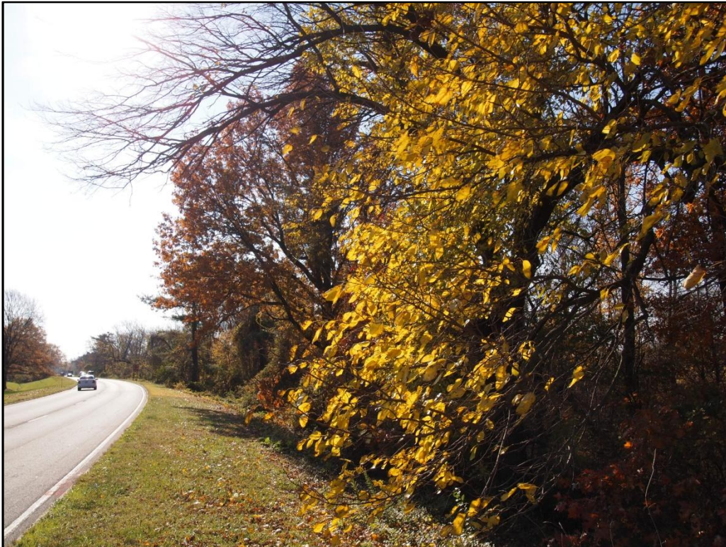
Plate 9: View southbound on the MVMH/PNCR showing area where a portion of the vegetation would be removed for the construction access road proposed as part of Build Alternative B.
