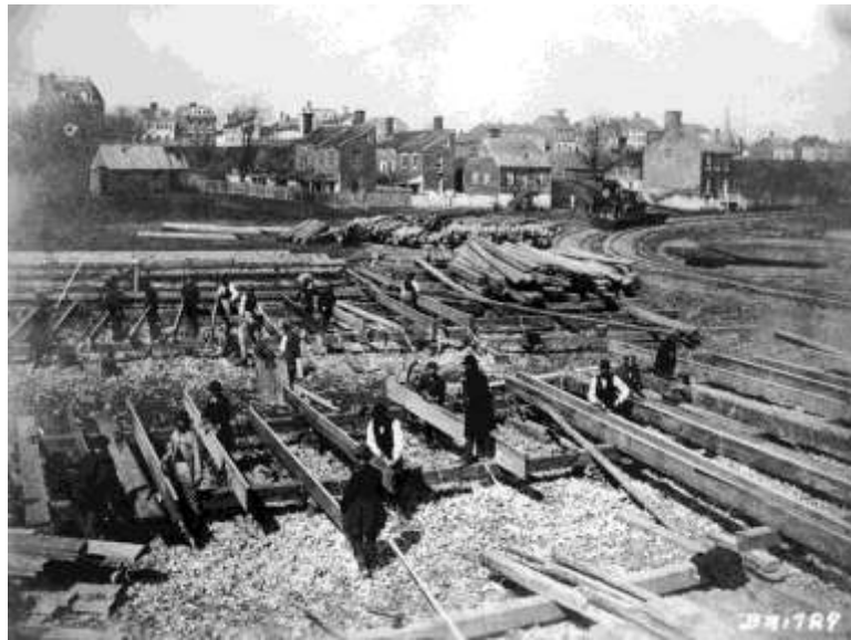
Workers of the USMRR probably assembling bridge trusses at the foot of Franklin Street, ca. 1863 Library of Congress
