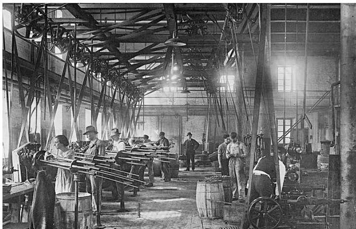
The Express Spark Plug Factory (shown here in the 1920s) replaced the Mount Vernon Cotton Factory at 515 N Washington Street (courtesy of Alexandria Local History Special Collections)
