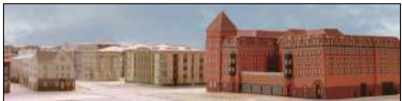
Figure 3. View of Fire Station from Main Street
