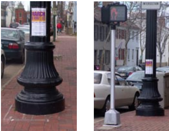
FIGURE 4.27 - Pole out of scale with the size of the sidewalk FIGURE 4.28 - Inappropriate mix of pole infrastructure
