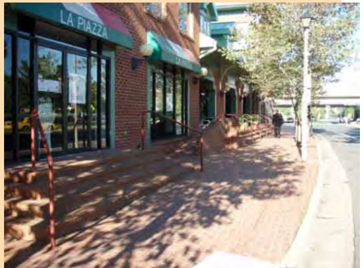
Retail space in the Colecroft building
