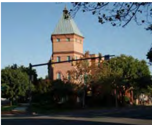
Building elements that rise above the context of surrounding buildings should be treated as attractive landmarks.
