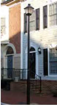
Dominion Virginia Power colonial light fixtures
