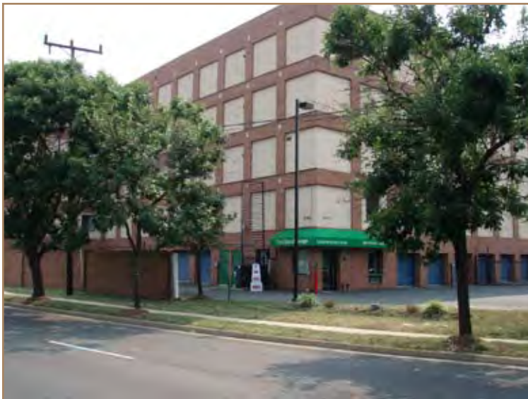
Early 20th-century warehouse building along Fayette Street
