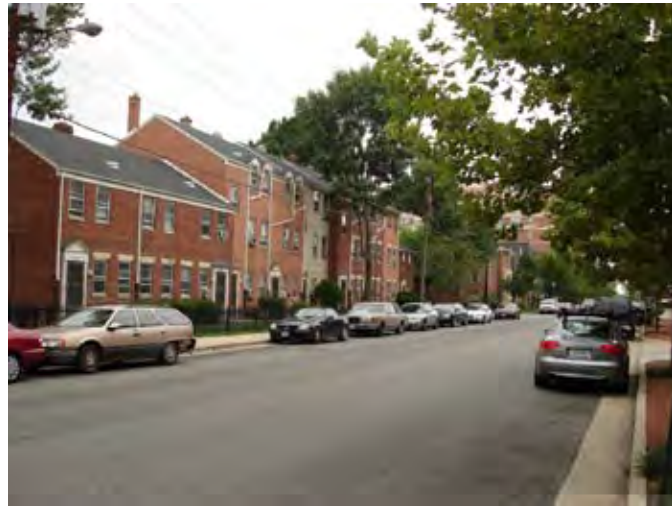
Two- and three-story townhomes units at the Andrew Adkins public housing site.
