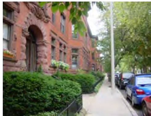
This building incorporates high quality brick with heavier masonry materials at ground level.
