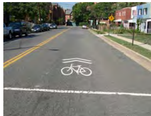
Existing "sharrow" pavement markings on Pendleton Street
