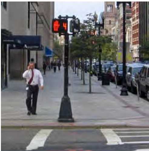
Countdown crossing signals alert pedestrians to the remaining safe crossing time more effectively than simple flashing signals.
