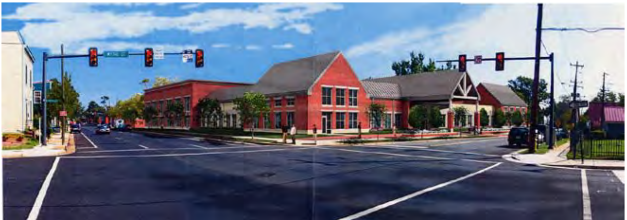
The soon-to-be-completed Charles Houston Recreation Center is aiming for LEED Silver certification.
