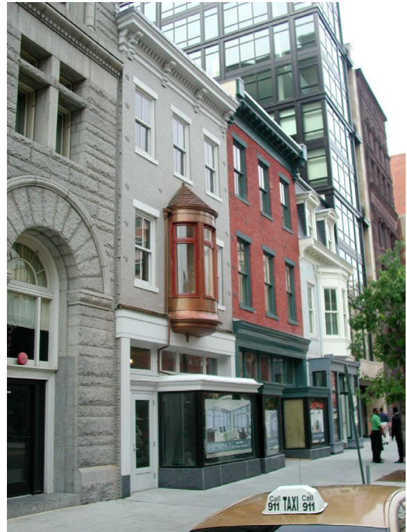
A series of facades resembling separate buildings helps reduce the perceived mass and scale of these building.
