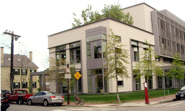
This building makes a transition to an adjacent residential street by terminating in a smaller building mass that matches the scale of nearby houses.
