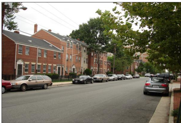
Two- and three-story townhomes units at the Andrew Adkins public housing site.
