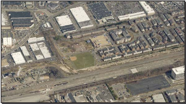
Neighborhood context. The Norfolk Southern tracks and Cameron Run separate the site from uses along Eisenhower Avenue, shown at bottom right in this photo. Pickett Street runs along the upper left. The Cameron Station residential development is to the right of the school.
