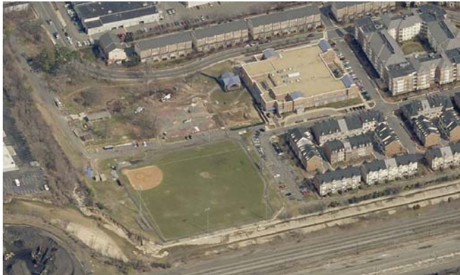
School site looking north, showing adjacent park and ball field. Cameron Run runs along the lower part of this photo.
