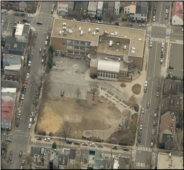
School site looking south across Wilkes Street with St. Asaph Street on the right of the image
