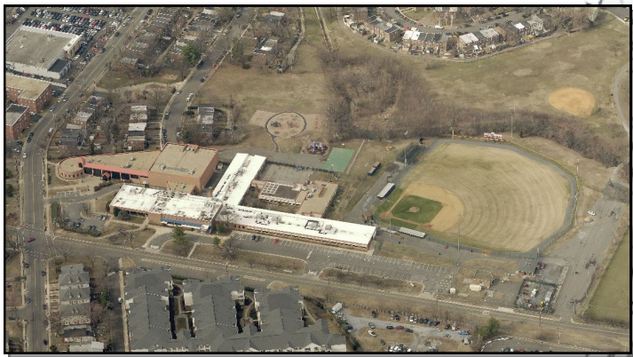
School site looking west across Commonwealth Avenue
