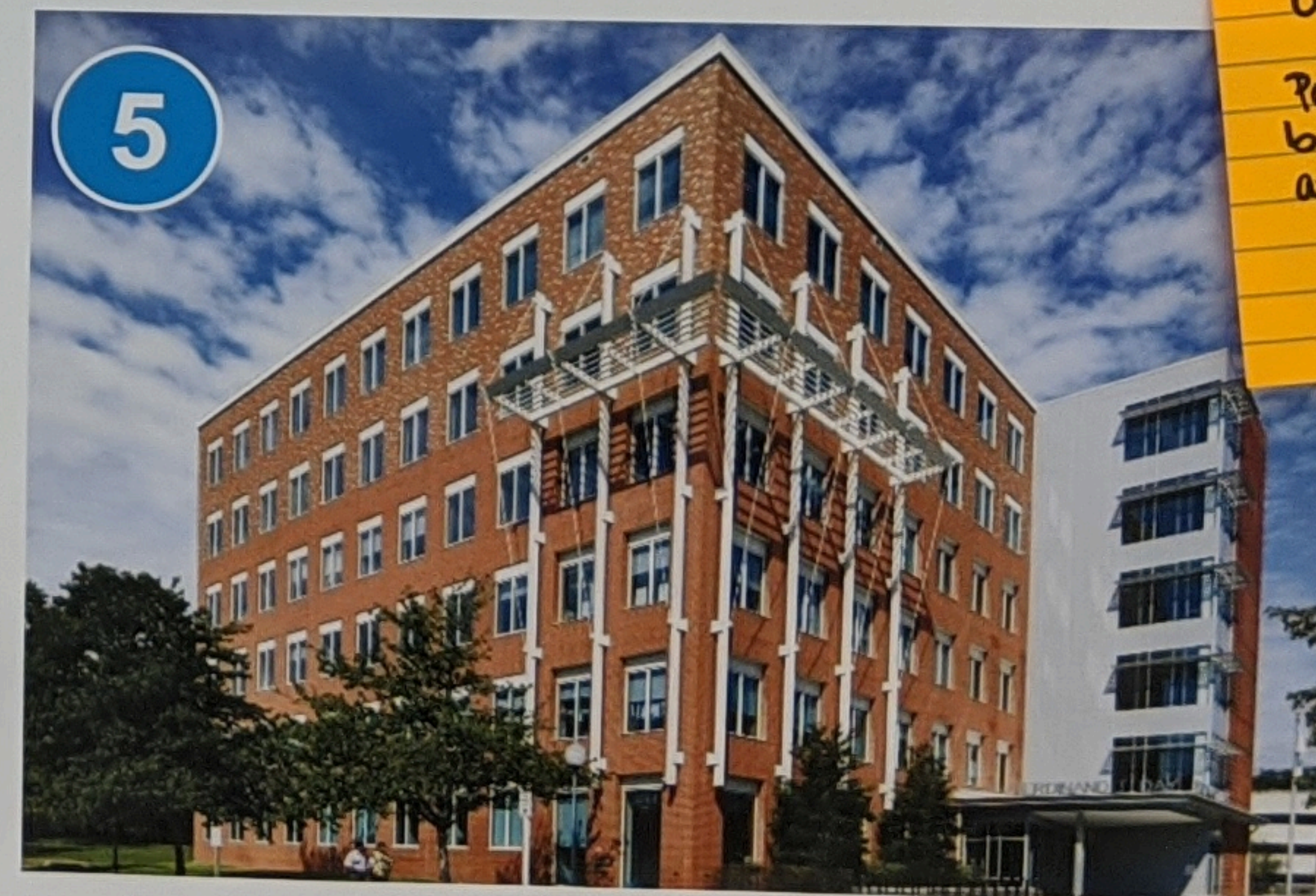
5 Ferdinand T. Day Elementary School Adaptive Reuse of Office Building – Elementary School & Future ACPS Admin Alexandria, VA
