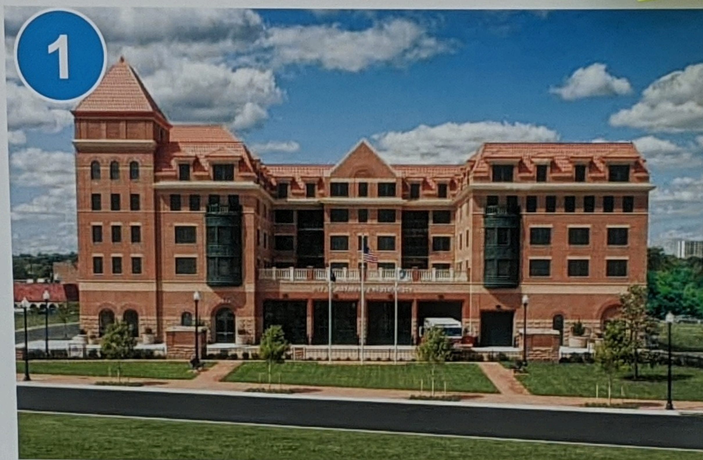
1 Potomac Yard Fire Station Colocated Fire Station with Affordable Housing Alexandria, VA
