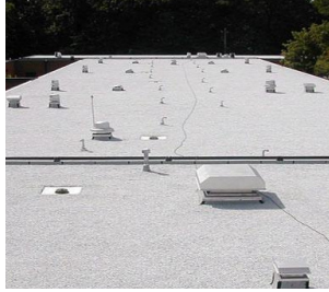
Built-Up Roofing (EPDM, TPO)
